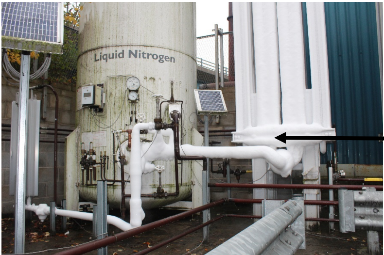
Fig. 3.9 Photograph of the cryogenic liquid N 2 routed via a vaporiser prior to the GMS [110].
