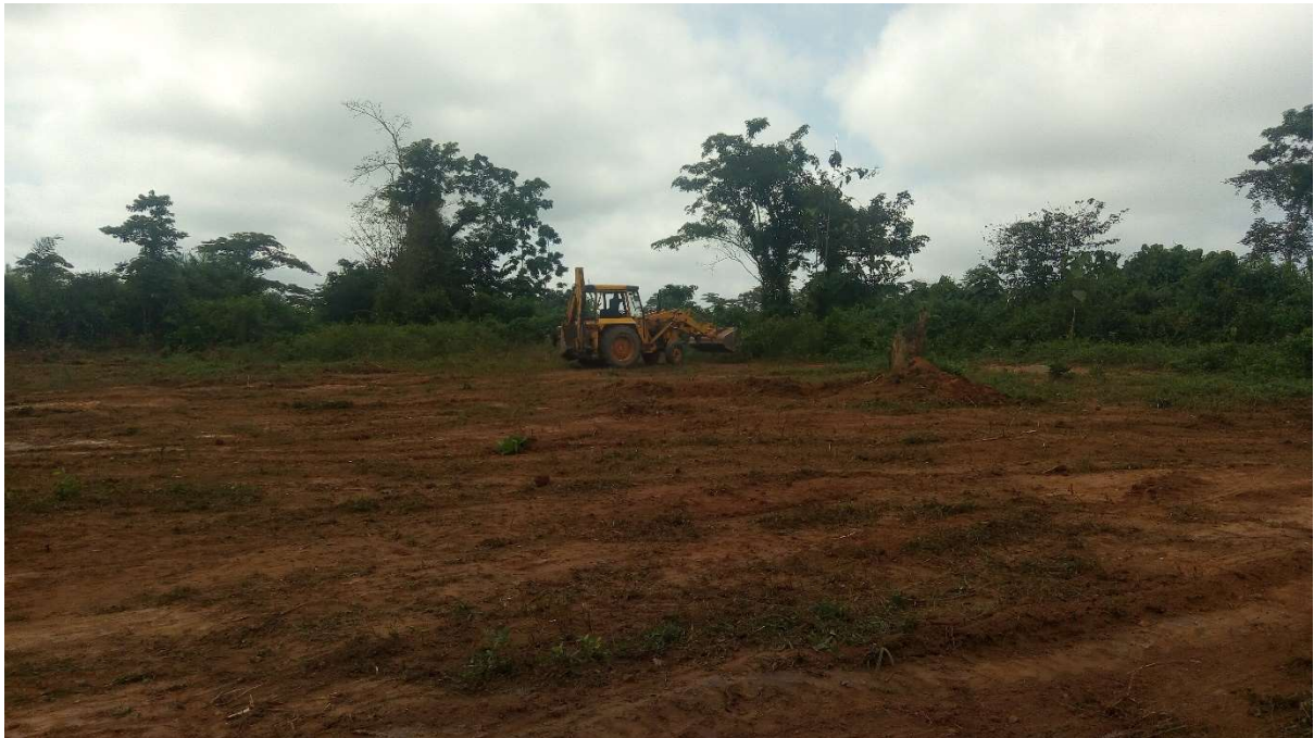
Pic 7.9 Clearing of the Land for the Outpatients Department Structure
