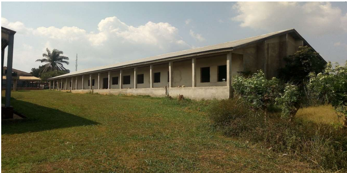
Pic 9.6 The Abandoned Children's Ward project at Mampong General Hospital
