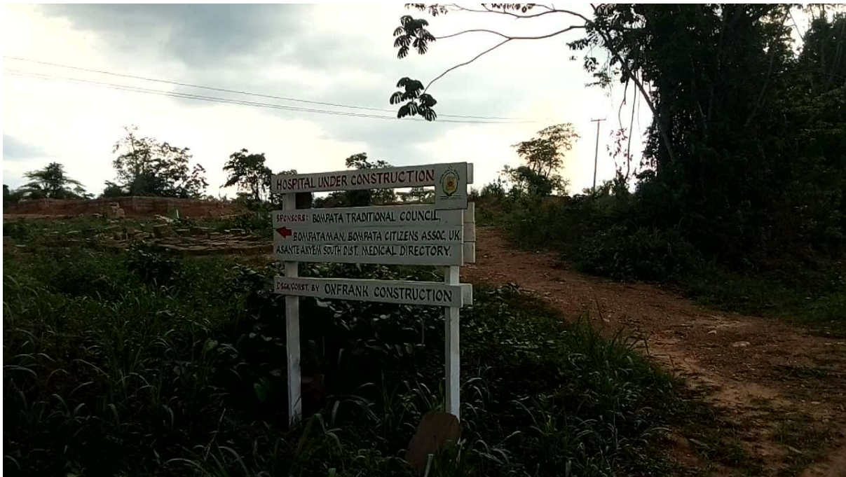
Pic 9.5 The New Hospital under Construction on the outskirts of Bompata
