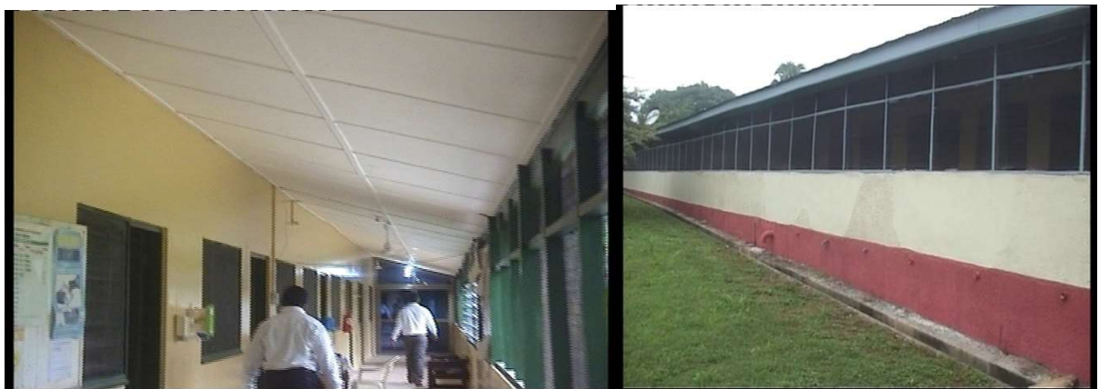
Pic 7.6 Pictures of the Refurbished Antenatal Ward
