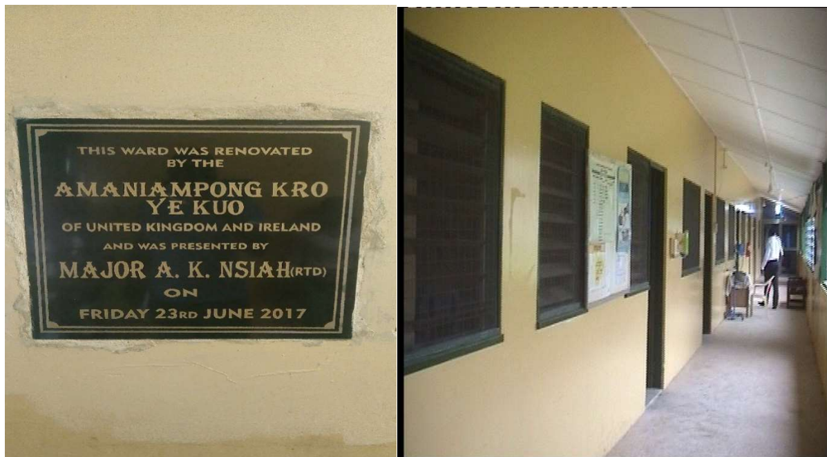
Pic 9.7 The Renovated Antenatal Unit at Mampong General Hospital in Mampong
