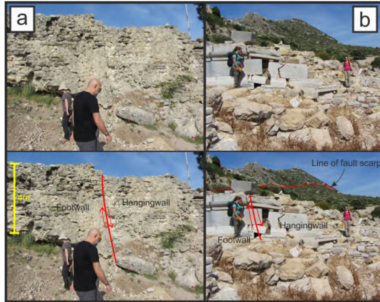
Figure 1.8: a) A 1st century aqueduct offset in a normal sense by the Manisa fault and subsequently repaired (N38.616647N, E27.319535). b) An offset temple in the ancient city of Knidos, western Turkey (N 36.688903, E 27.373262). The responsible fault is seen in the form of a limestone fault scarp in the background. The offset can be traced through the ancient ruins.
