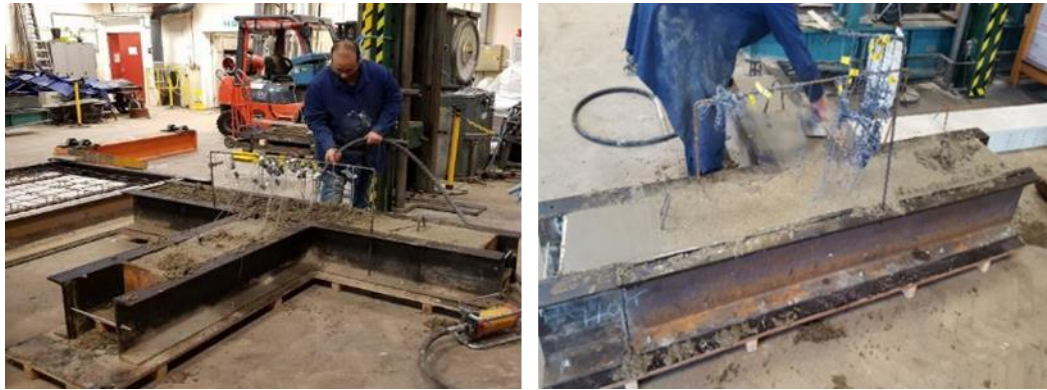
Figure 3.6: Casting using the hand-held vibrator
