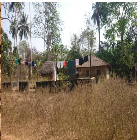
Fig. 28 A house destroyed by fighting during the war is now used to dry clothes. Bauya, Sierra Leone Source: Author 2017.
