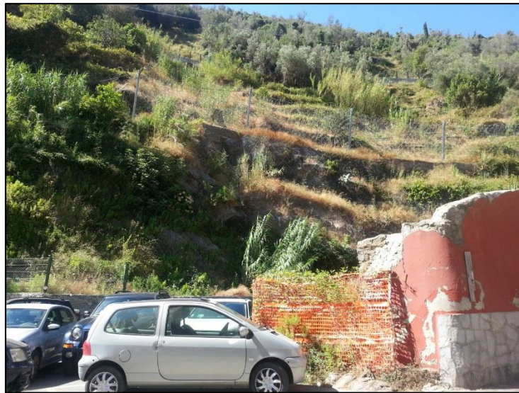
Fig. 30. Vernazza. Structural flood damage, far away from the tourist gaze. Photograph by author.
