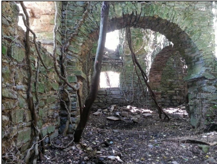
Fig. 46. An abandoned drystone building near the landmined area. Photograph by author.
