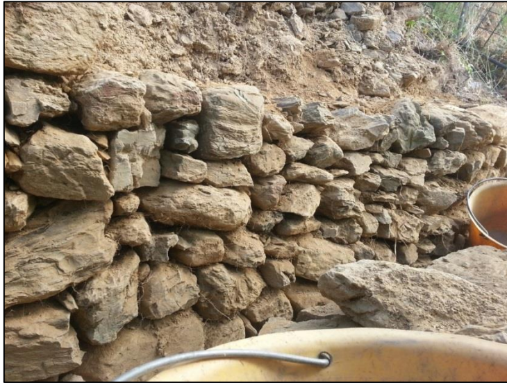
Fig. 51. Vernazza. A freshly laid drystone wall. Photograph by author.
