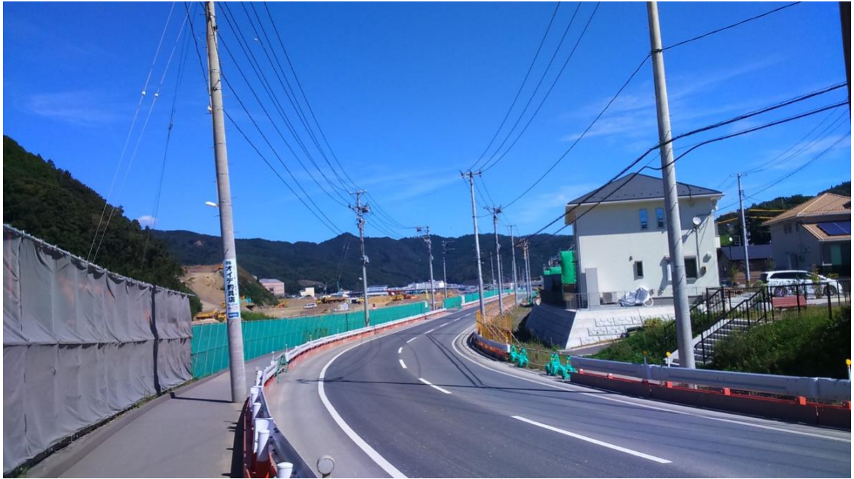
Image 4: Post-disaster infrastructure in Onagawa, Anna Vainio, September 2016
