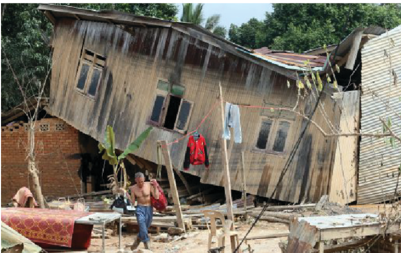
Figure 5.20 The house washed away during flooding (Source: Ibnuhasyim, 2015)
