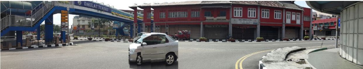
Figure 4.11 (View 2) Old shop lots built in 1928 are still empty since the major flood in 2006/2007. Buildings were inundated up to the second-floor level.
