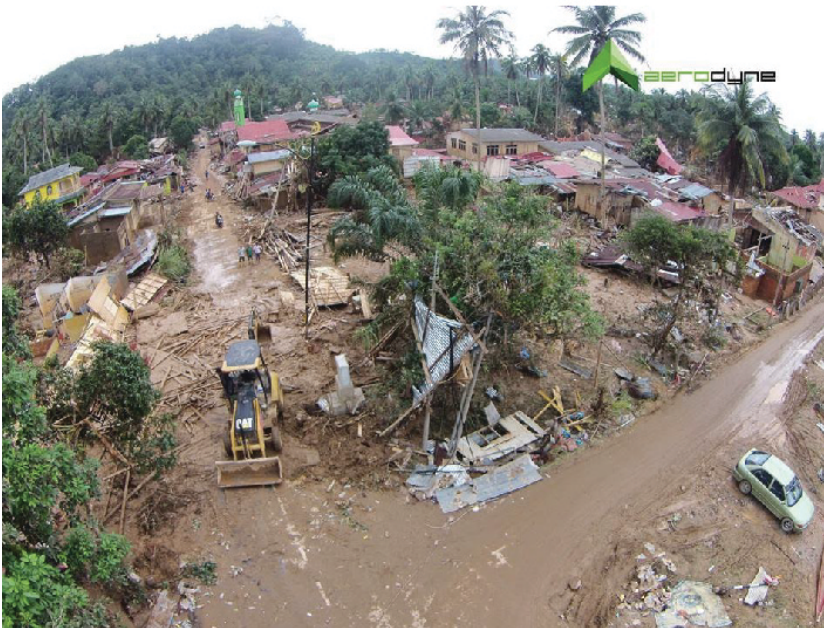
Figure 5.13 After flood disaster clearing and cleaning process (Source: Bharian, 2014)
