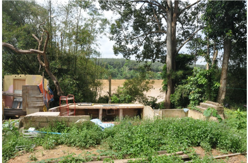
Figure 5.34: The condition of a house in Kampung Hujung Tanjung, near the Lebir River (behind with brownish water) that was destroyed and washed away during the flood. It is now left with ruins of the kitchen area constructed out of bricks. Picture taken on 16th December 2015 from KL's house entrance staircase (Nor Izura T., 2015).
