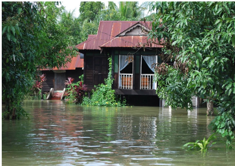
Figure 2.19 (above) The on-stilts features allow room for daily activities including parking boats underneath the house (Source: Malaysian Timber Council, 2018)
