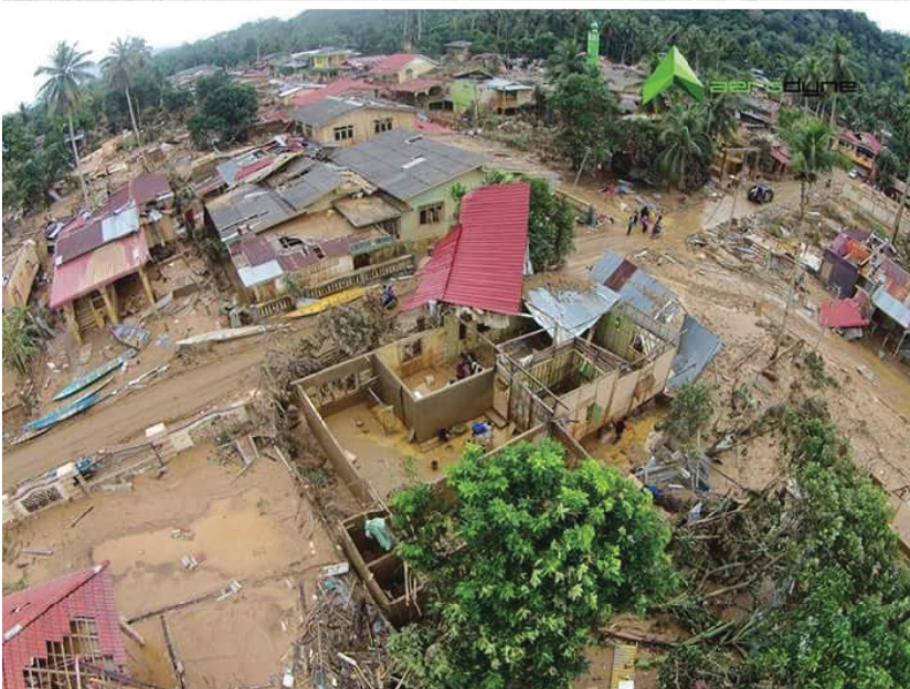
Figure 5.14 An overview of after flood disaster in one of the kampung in Kuala Krai. Roads and houses were severely covered with thick mud. (Source: bharian, 2014)
