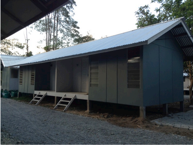
Figure 5.28 Transit house initiated by Mercy Malaysia for 30 families. This development includes common toilets, common kitchen and a multi-purpose space (Nor Izura T., 2015).
