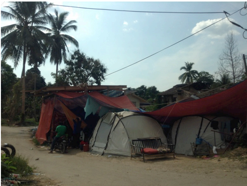
Figure 5.25 & 5.26 Temporary shelters donated by ShelterBOX for flood victims in Kuala Krai. Victims have stayed in the tent for more than a month. A layer of canvas on top of the tent functions as a double-layered roof due to the hot and humid weather especially during the day. (Nor Izura T.,2015)
