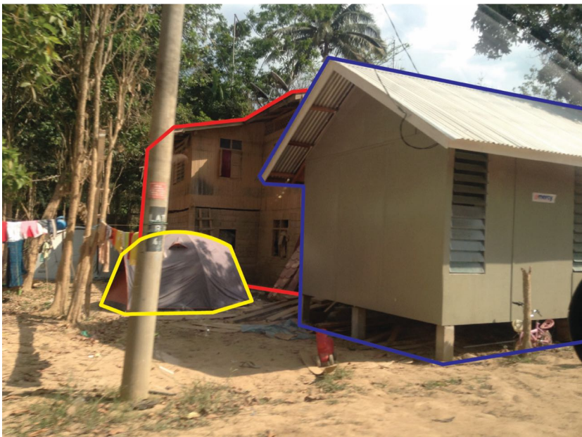
Figure 6.6 Picture shows the situation people (from PMT) been through during transit. The house highlighted in red was the original dwelling, which could not be occupied anymore due to damage. After coming back from the relief centre, the residents were provided with temporary shelter highlighted in yellow (funded by various agencies). They were then relocated to a transit house (highlighted in blue) after 3 months living in the shelter.
