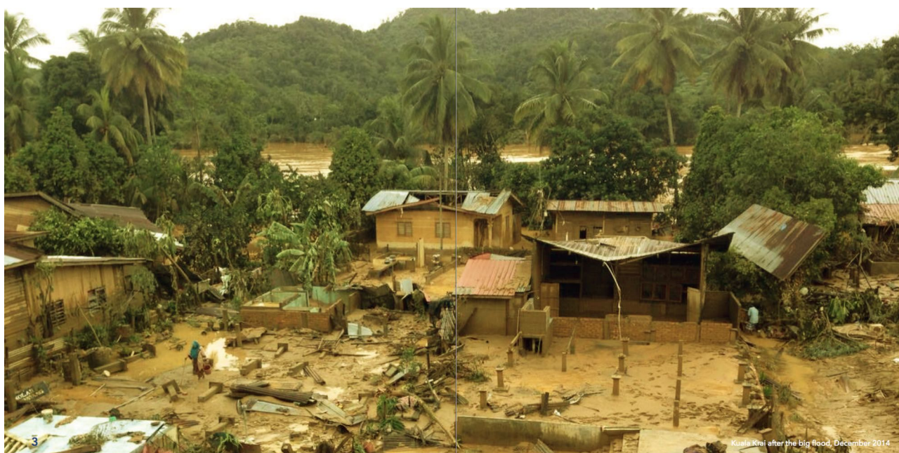
Figure 5.8 View after the flood disaster. Houses were damaged severely, and covered with thick mud (Source: Mercy, 2016)
