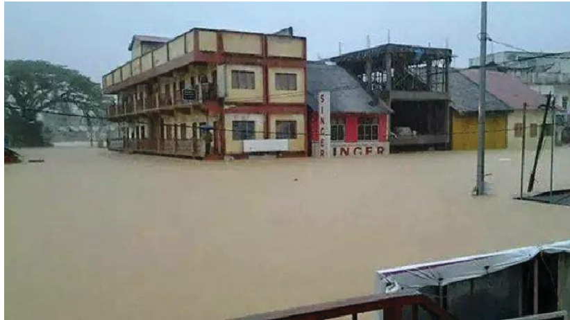
Figure 5.15 Flood rose up to 3 metres height and affected the shoplots and houses at Kuala Krai town. (Source: mstar, 2014)
