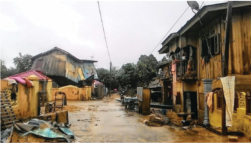
Figure 5.12 A house (on the left) was washed away by the flood and stuck on top of another house (Source: bharian, 2014)
