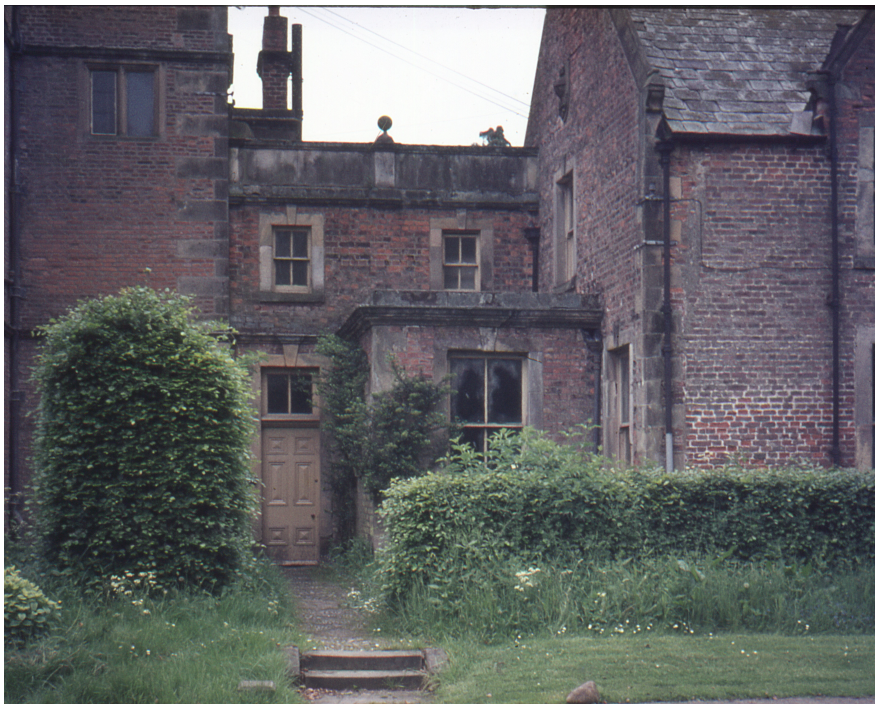
Figure 3.28: Kiplin Hall 'housekeepers link' in 1976 (Kiplin Hall Trust)
