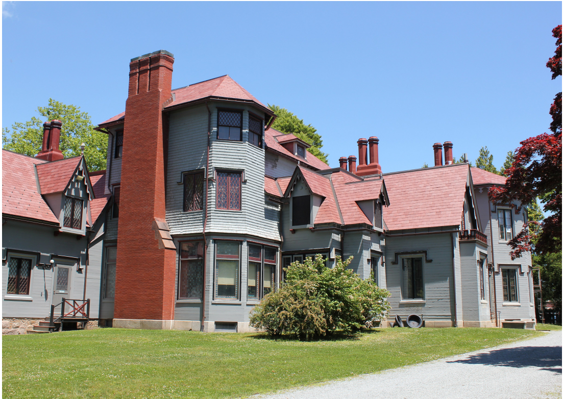
Figure 5.5: Kingscote McKim, Mead and White addition (© Dms1788, cc by-sa/4.0)
