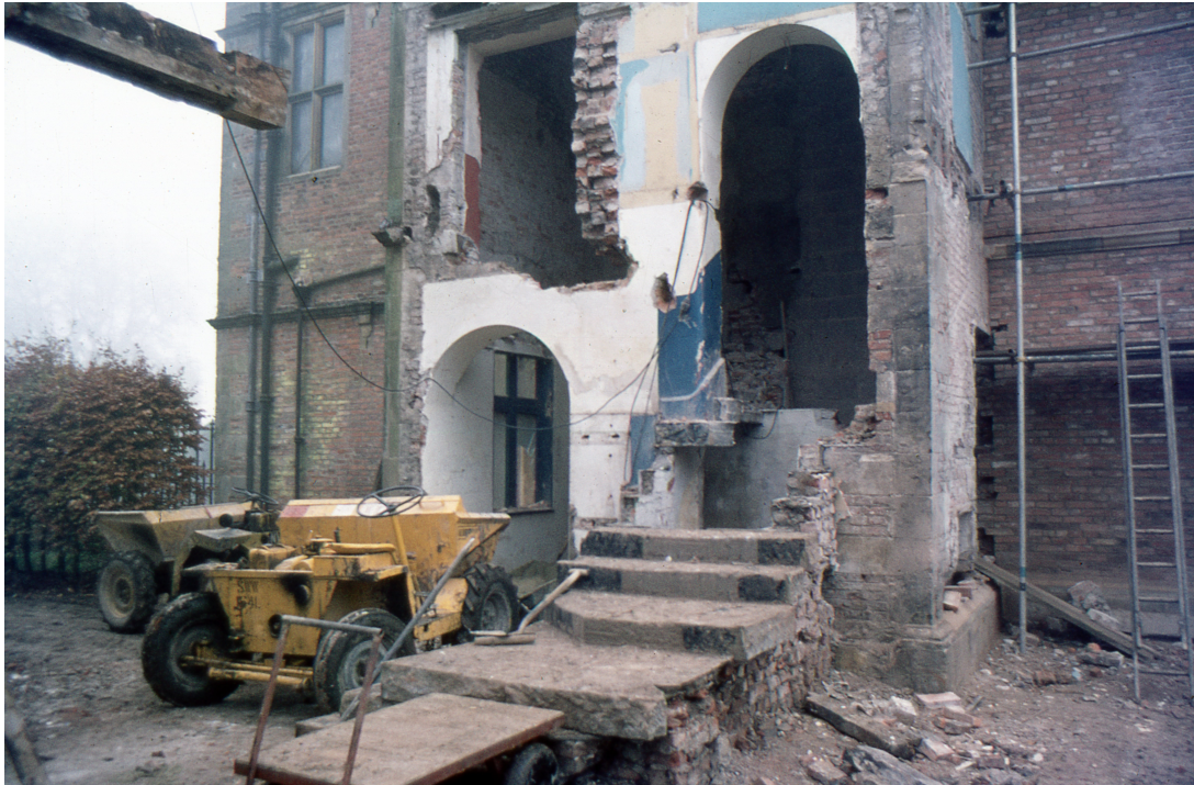
Figure 3.29: Kiplin Hall north tower staircase demolition 1976 (Kiplin Hall Trust)
