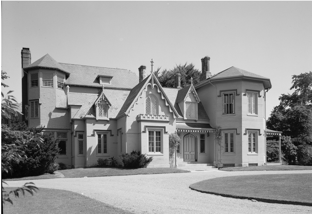
Figure 5.1: Kingscote from the southwest ( Historic American Buildings Survey, HABS No. RI-307 )
