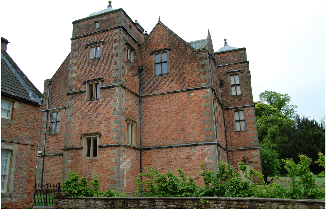
Figure 3.6: Kiplin Hall north façade and reconstructed tower
