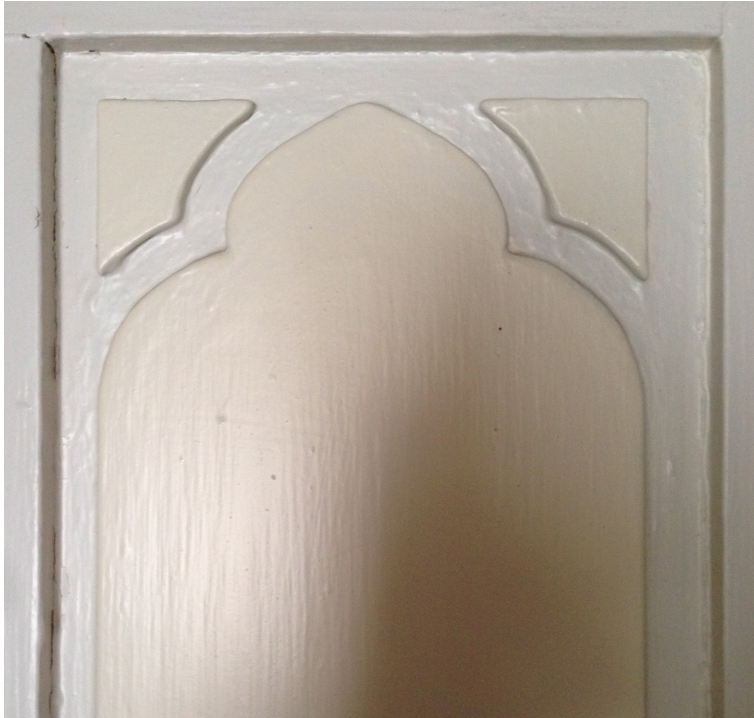
Figure 5.13: Kingscote servant door (detail)
