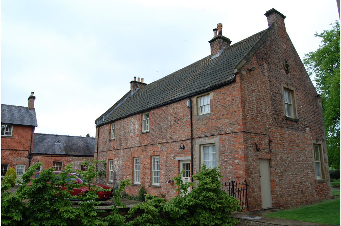
Figure 3.8: Kiplin Hall kitchens view from southwest
