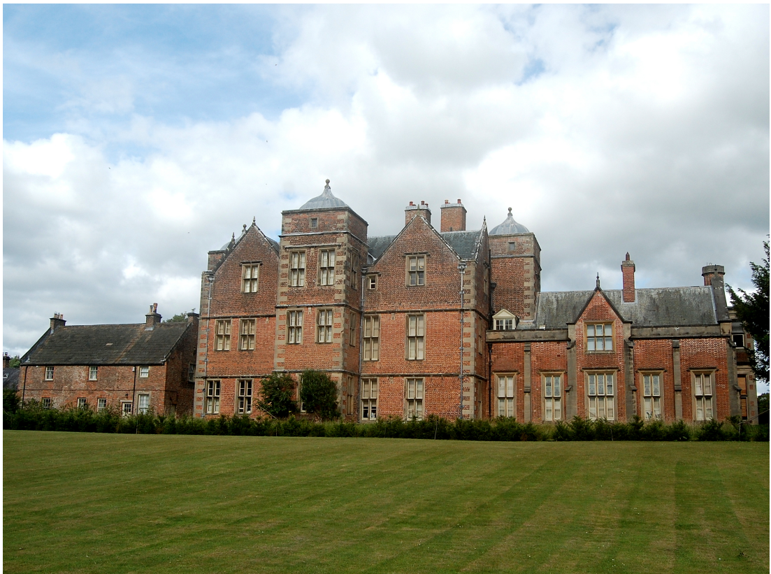
Figure 3.5: Kiplin Hall west façade (© Bill Harrison, cc-by-sa/2.0)
