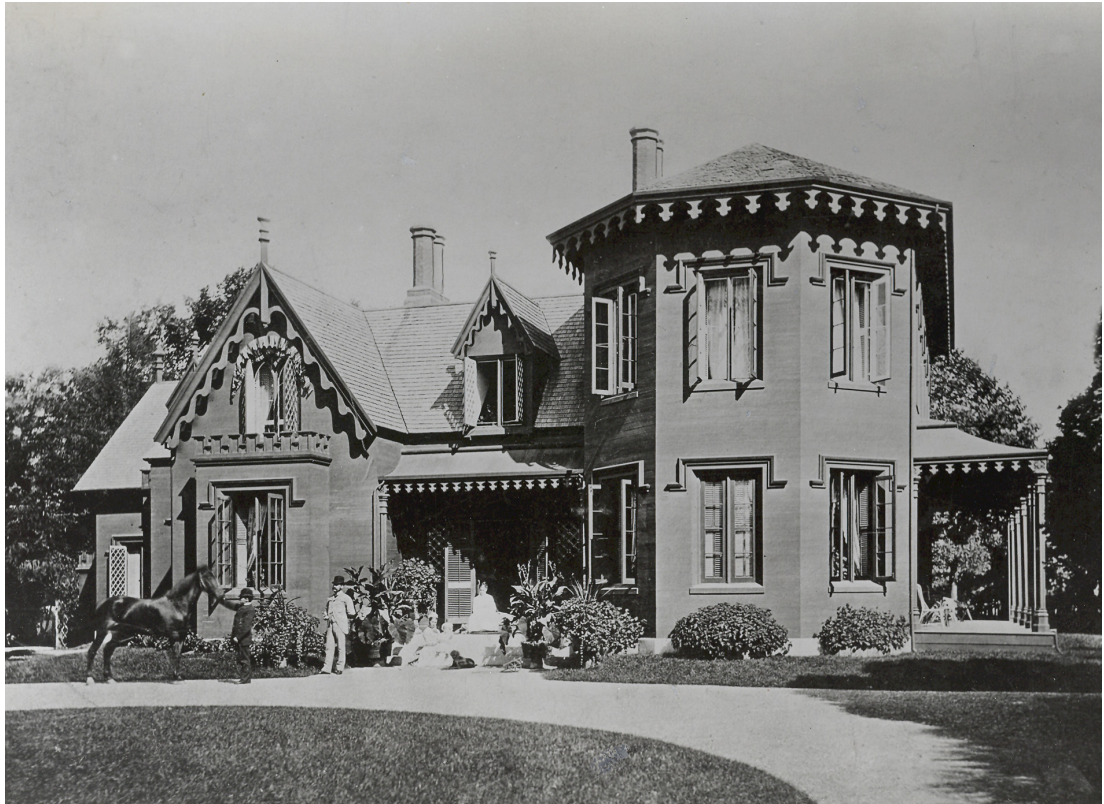
Figure 5.19: Kingscote 1878 south elevation, laundry addition left (from the collection of The Preservation Society of Newport County)
