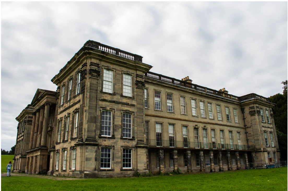
Figure 2.17: Calke Abbey east façade (© Oliver Mills, cc-by-sa/2.0)
