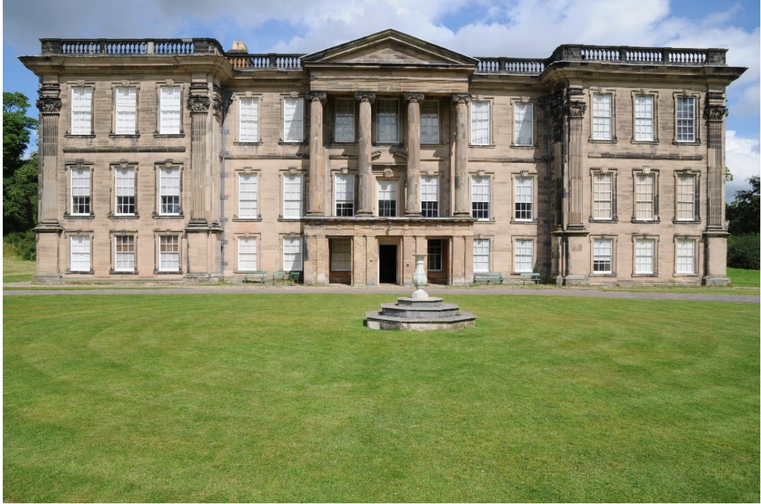
Figure 2.18: Calke Abbey south façade (© Philip Halling, cc-by-sa/2.0)
