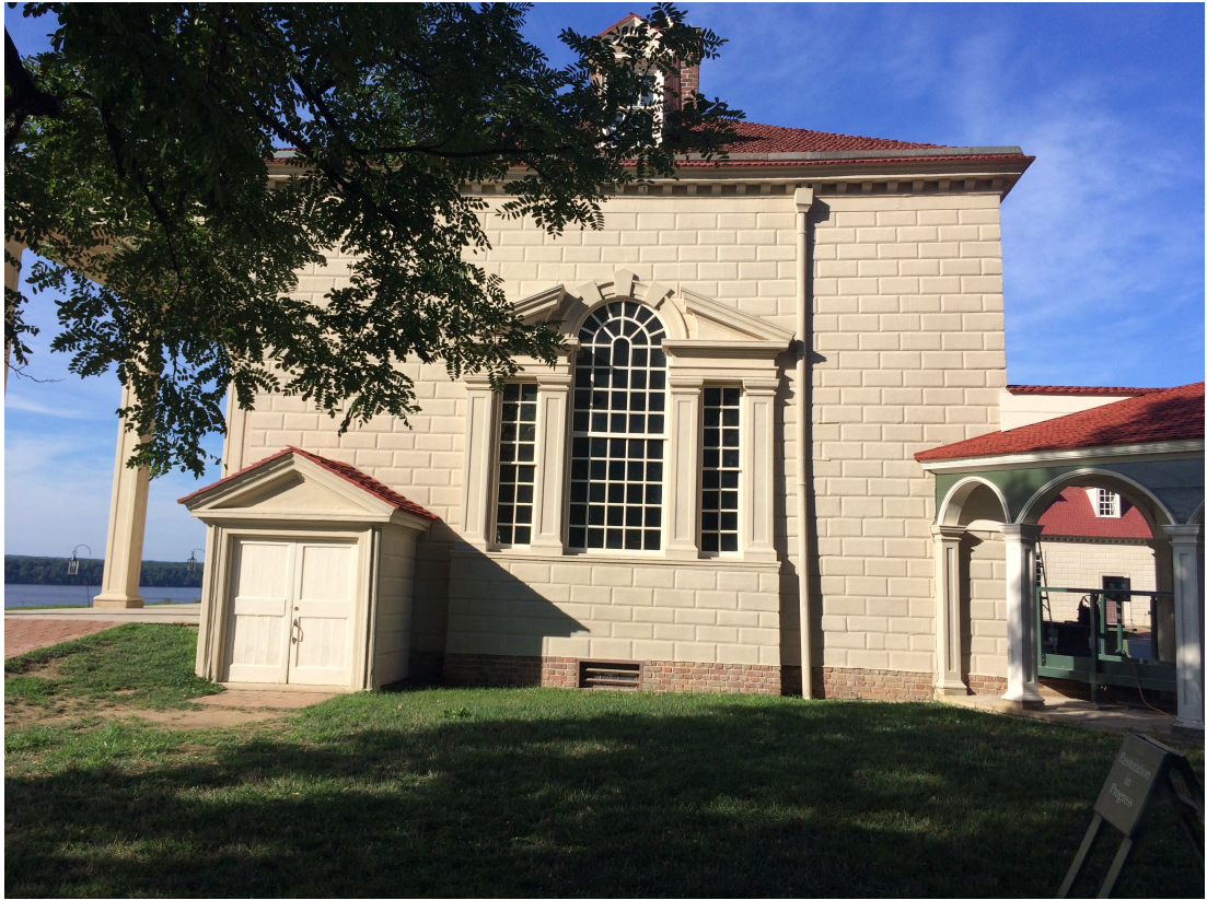
Figure 4.2: Mount Vernon Mansion north façade, Palladian window
