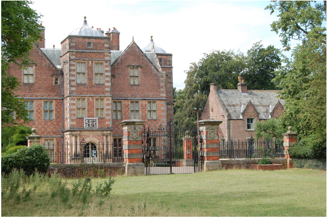
Figure 3.1: Kiplin Hall from the east
