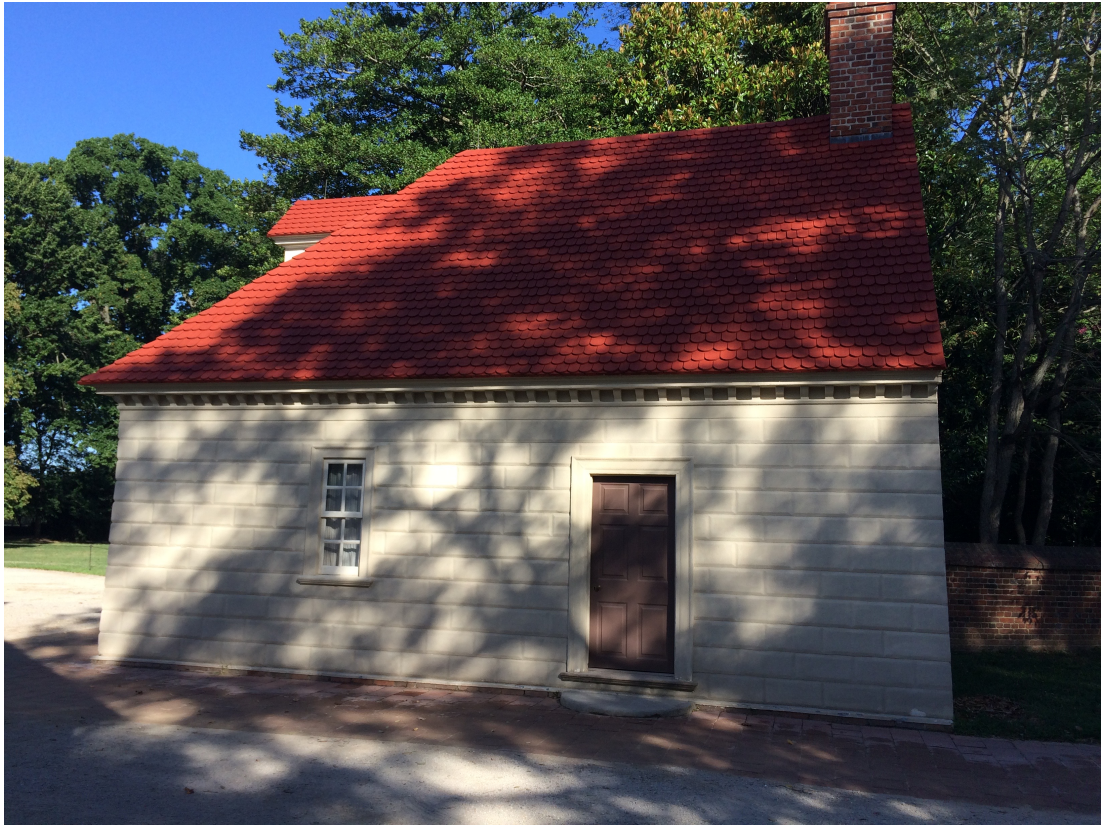
Figure 4.8: Mount Vernon gardener's house east side with half-hipped and half-gable roof
