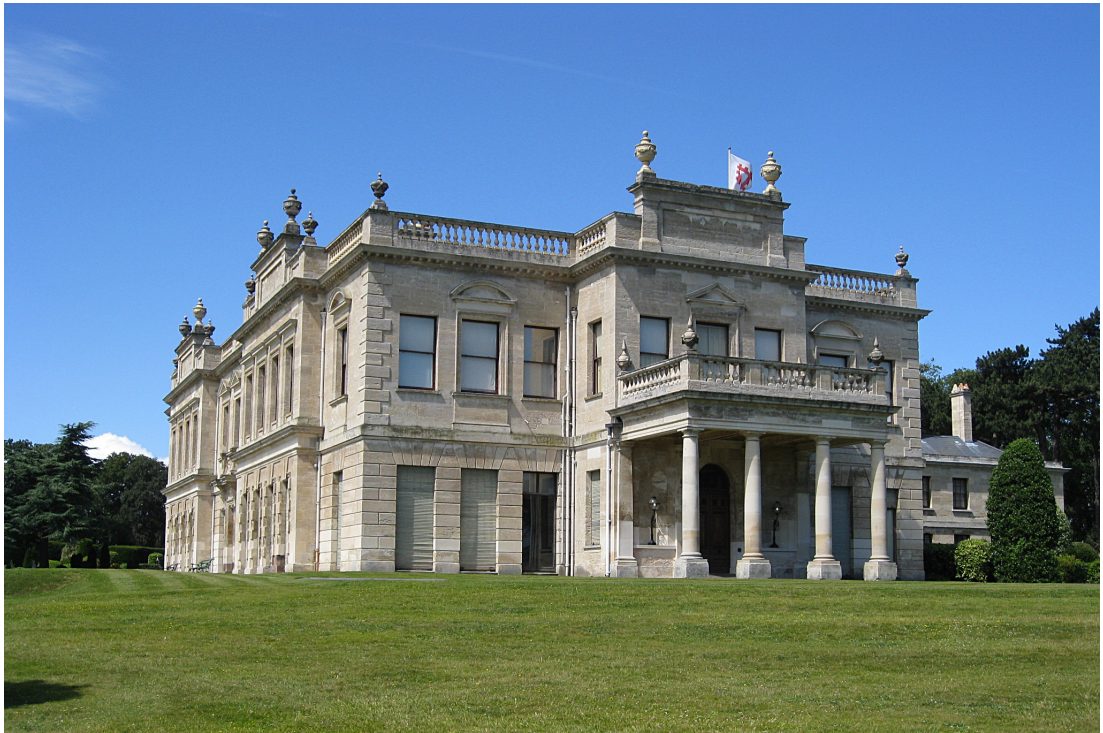
Figure 2.24: Brodsworth Hall east side (© Tony Bacon, cc-by-sa/2.0)
