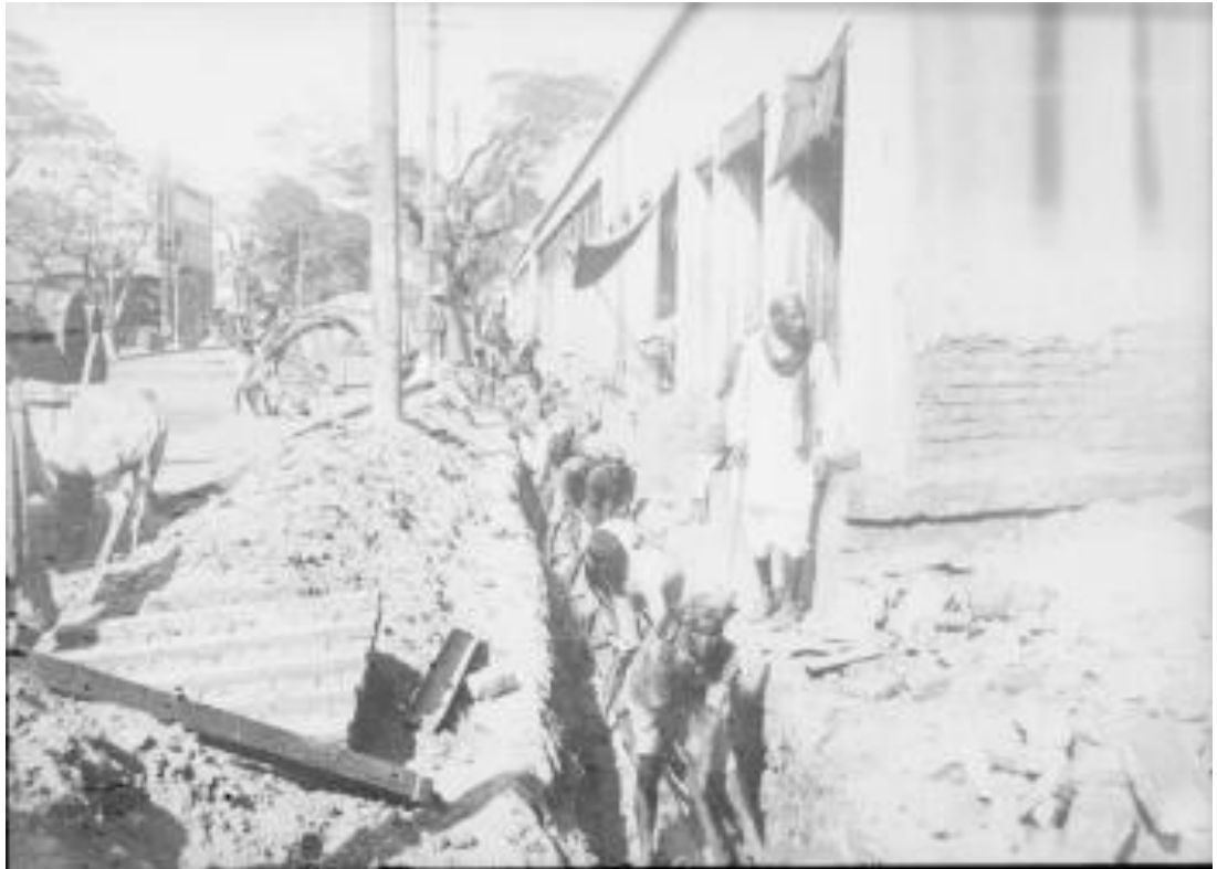
Figure 5.4: “Works photographic negative of cable laying, Calcutta: Shows cable being laid in trench by business premises.” W T Glover & Co. Ltd, 1900 - 1910 [Science and Industry Museum Manchester Archives YA1972.36/MS0231/Neg 258]
