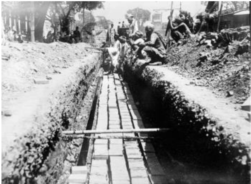
Figure 5.3: “Works photographic negative of trench, Calcutta: Shows trench with troughing with local men.” W T Glover & Co. Ltd, 1906 - 1916 [Science and Industry Museum Manchester Archives YA1972.36/MS0231/Neg 884]
