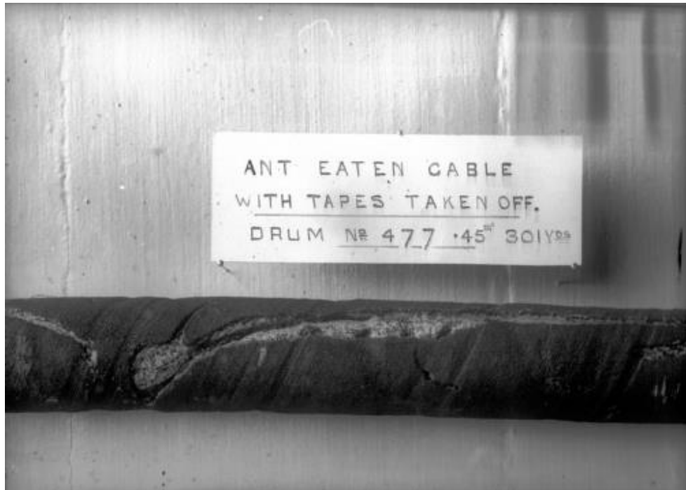
Figure 5.6: "Works photographic negative ant eaten cable, Calcutta". W. T. Glover & Co. Ltd, 1900 - 1910 [Science and Industry Museum Manchester Archives YA1972.36/MS0231/Neg 254]
