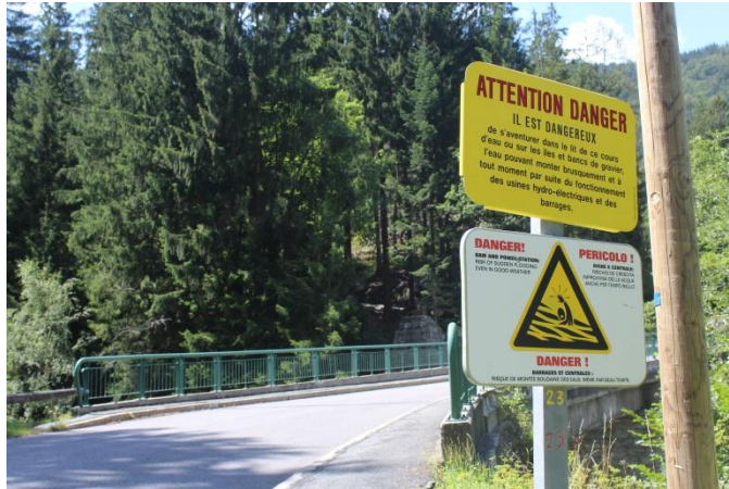
Figure 51 The Pont Pélissier with warning signs for flood release from hydroelectric dams
