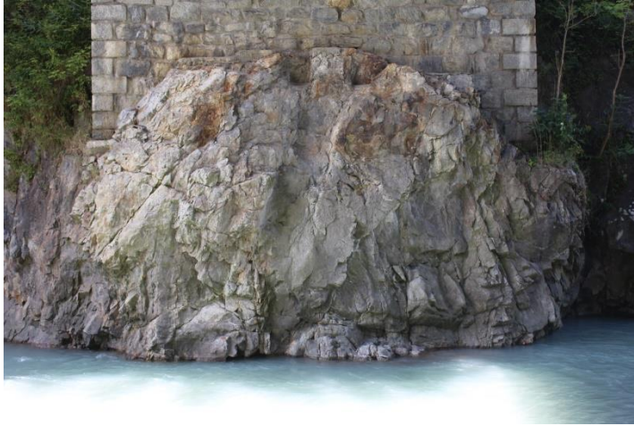
Figure 53 Span-beam housings at the top of the buttress for the low-level Pont Pélissier seen in eighteenth-century paintings and early nineteenth-century paintings.
