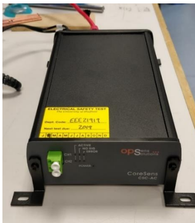
(a) General View of Fibre Optic system
