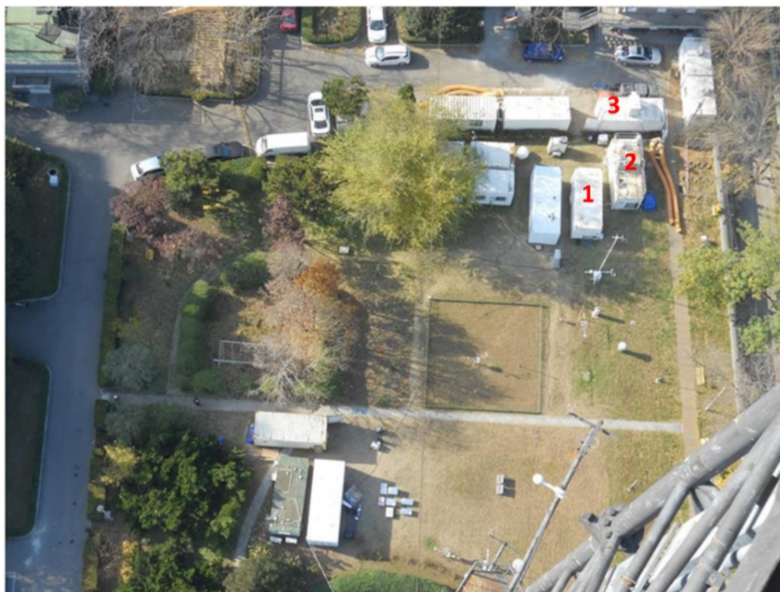
Figure 7.1 Picture of the Institute of Atmospheric Physics (IAP) showing the layout of the shipping containers housing different instruments. The container 1 housed the trace gas measurement ( O_3 , NO , NO_2 , CO ) as well as the VOC measurements. Container 2 housed the Leeds ground-based FAGE instrument used to measure OH , HO_2 , RO_2 and OH reactivity. Container 3 housed the PKU FAGE instrument that measured OH and HO_2 as well as trace gas measurements ( O_3 , NO , NO_2 , CO ). See Table 4.1 for detail on the instruments housed in each container.
