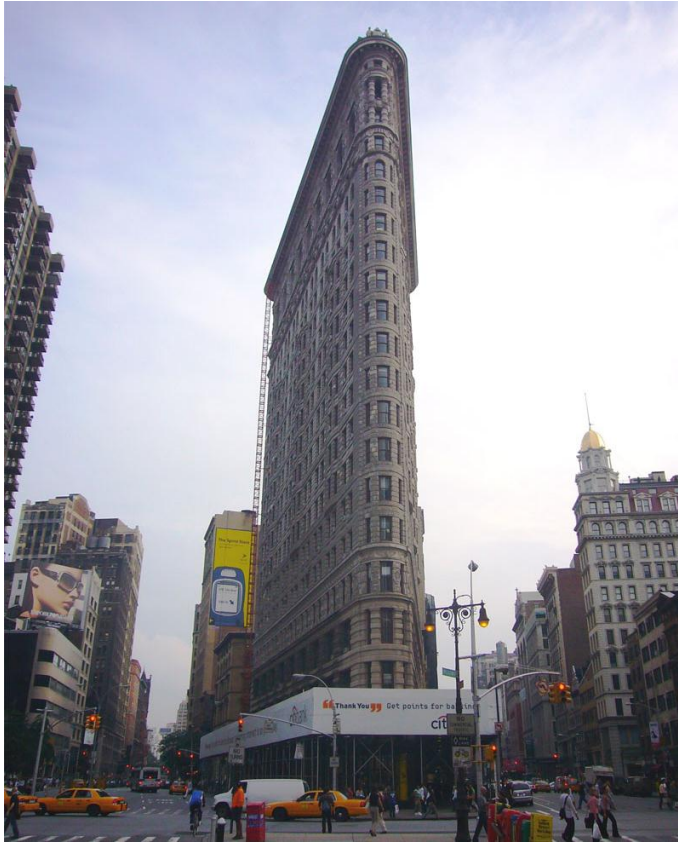
Figure 1.8: Flatiron building, New York
