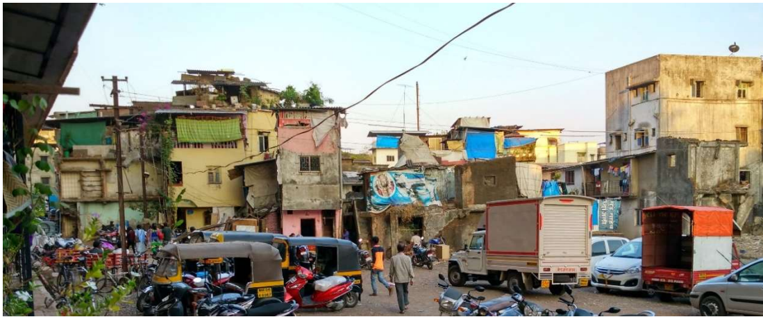
Figure 6-6 A side view of the settlement highlighting the multiple storeys high and semi-pakka and pakka structures (Source: Author’s own, 16 January 2016)
