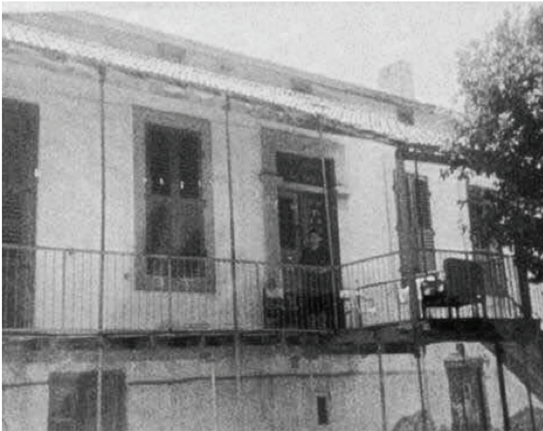
Figure: The front entrance to the Büyük Ev ; on the right side of the picture it can also be seen the locked door which led to the basement.
