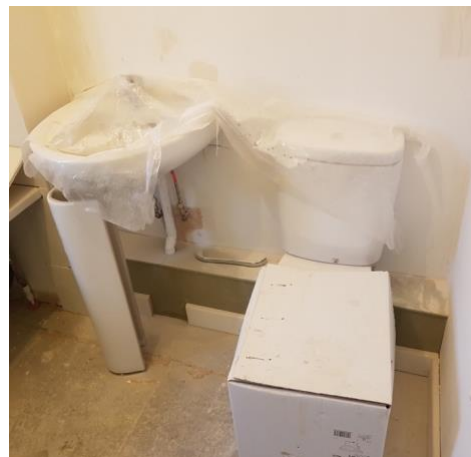
Figure 32: Photo of Construction Stage 7 (left)
