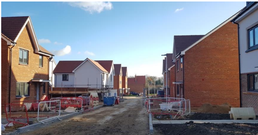
Figure 37: Photo of plots nearing completion
