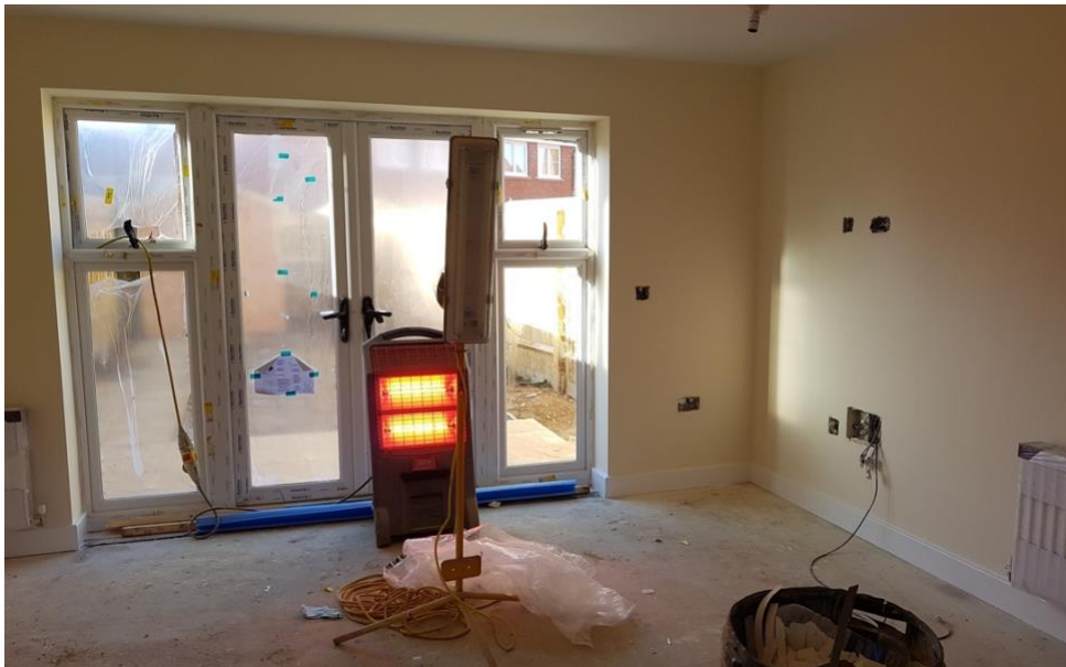
Figure 35: Photo of Construction Stage 10
