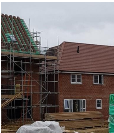
Figure 29: Photo of Construction Stage 5 (left)
