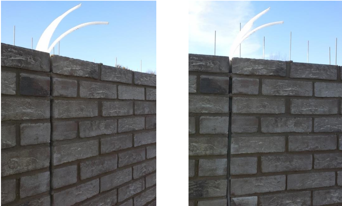
Figure 47: Photographs showing the vertical foam movement joint
