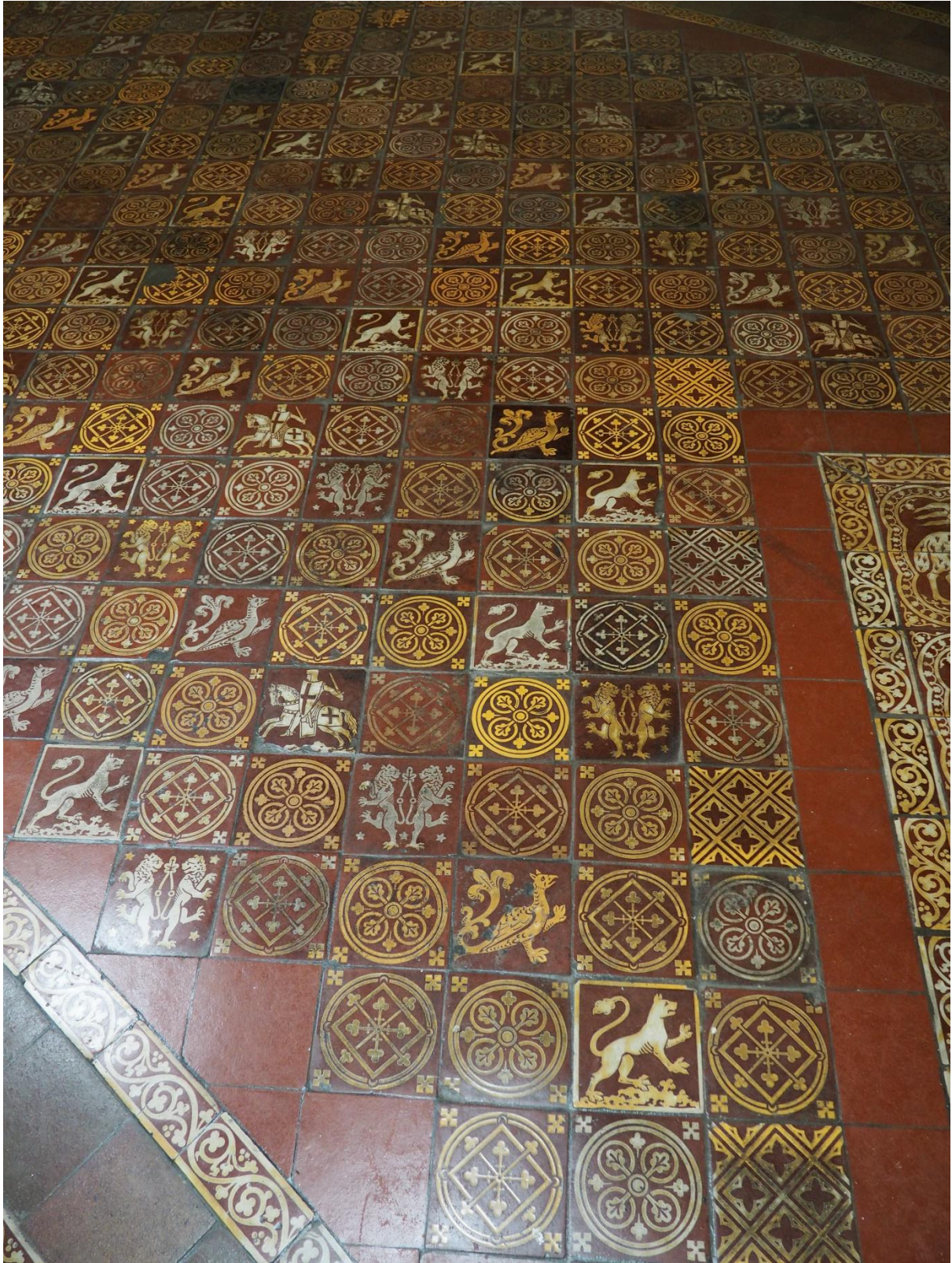
Figure 1.8 Temple Church: Minton tiles relaid in the rotunda triforium.
