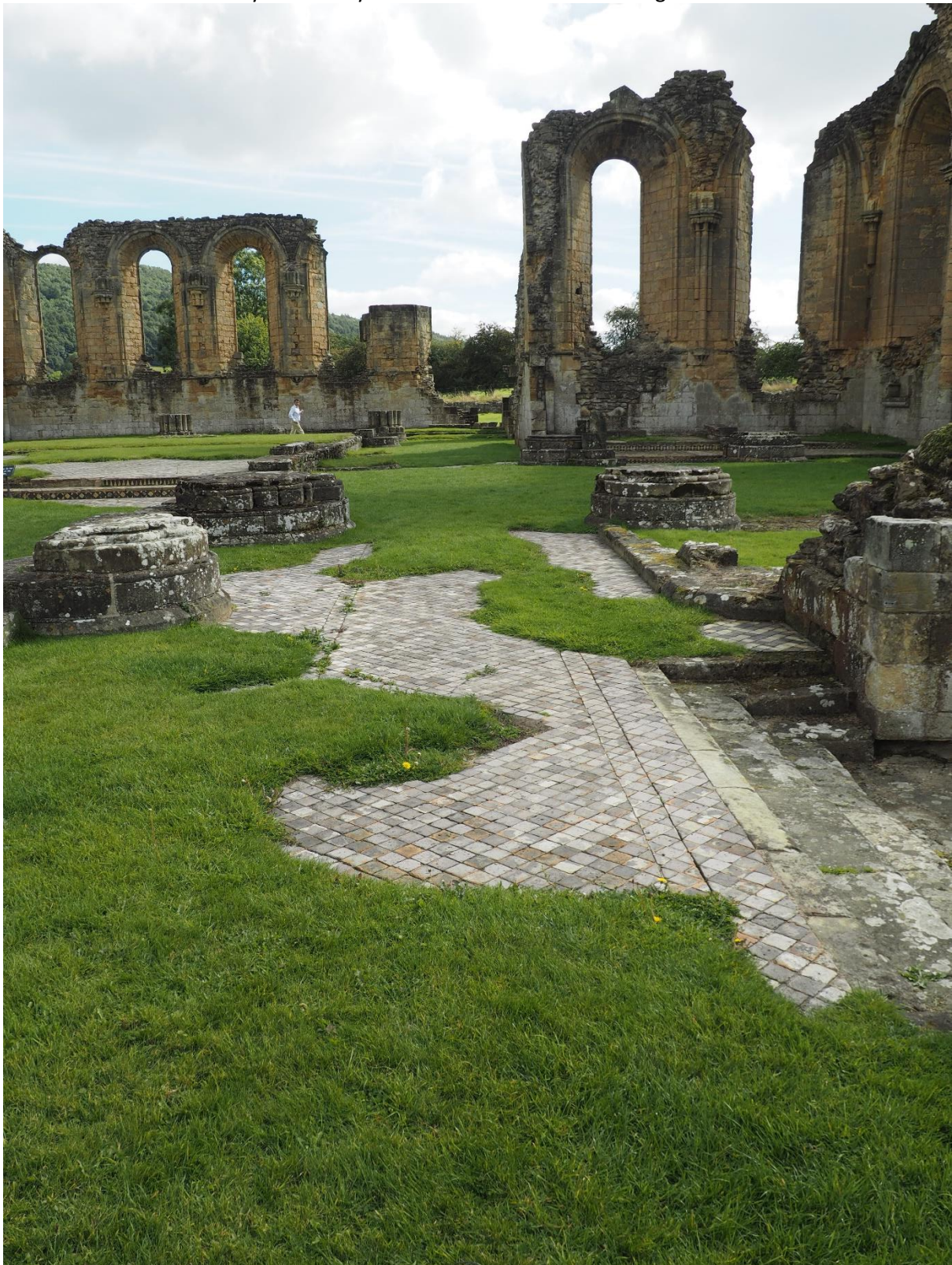
Figure 4.23 Byland Abbey: view of south choir aisle facing east.
