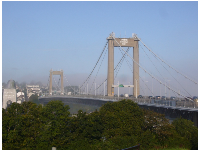
Figure 3.1: The Tamar Suspension Bridge
