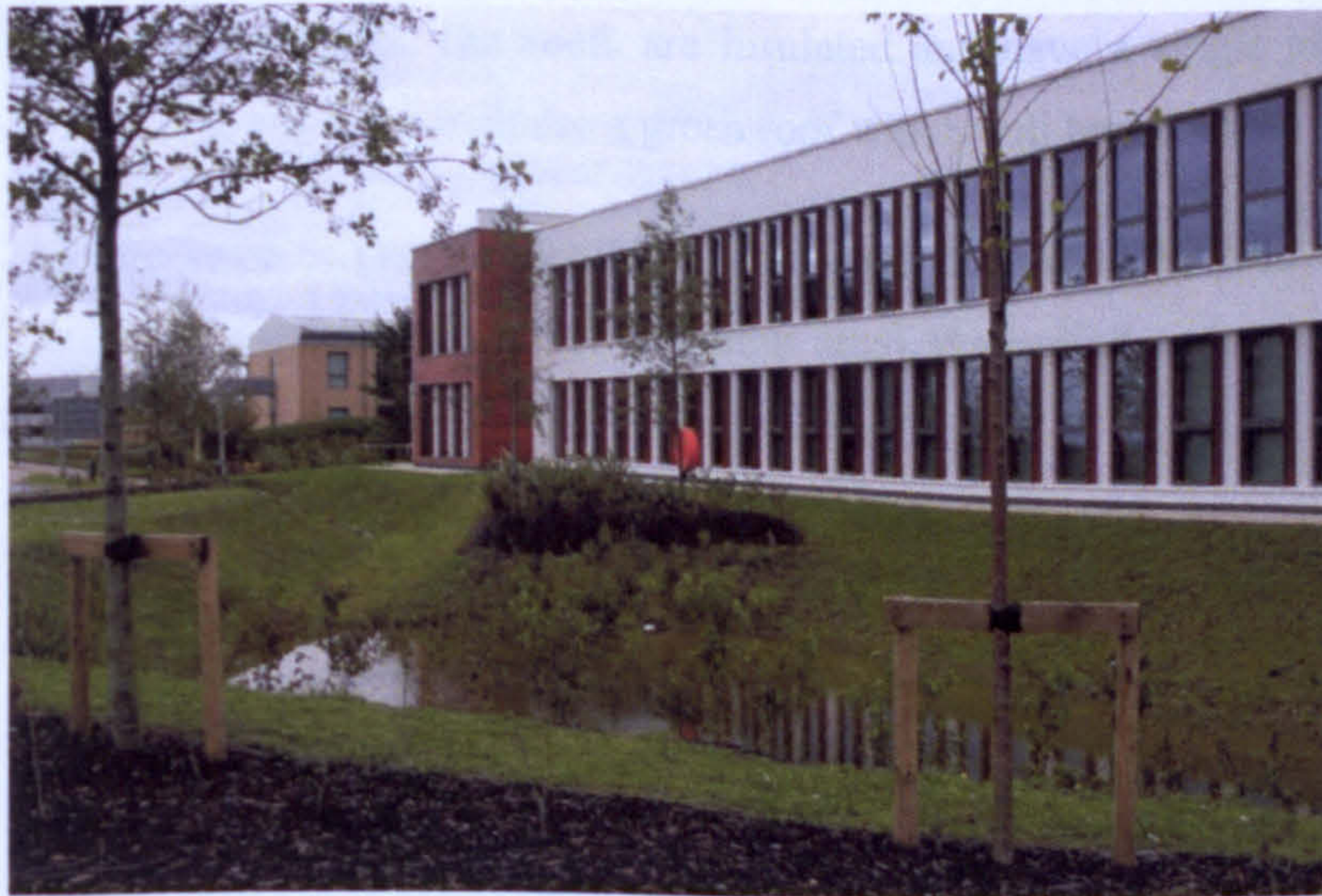
Figure 3-1: Case study office building
