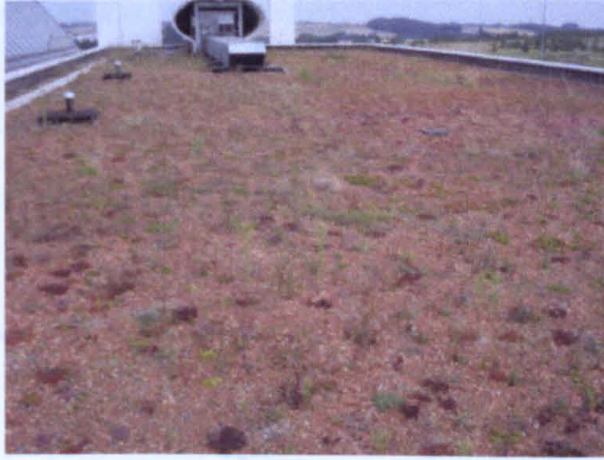
Figure 3-9: Sedum green roof on the roof of the east wing block
