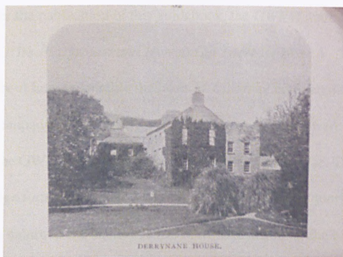
Figure 5.27. Derrynane House from Southern Ireland.
