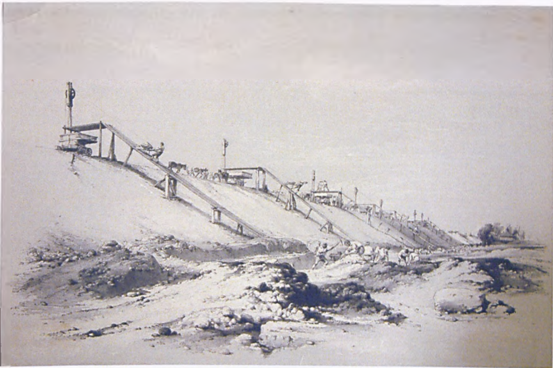
Figure 2.9. NRM 1900-004 (pt2). Box Moor Embankment.
