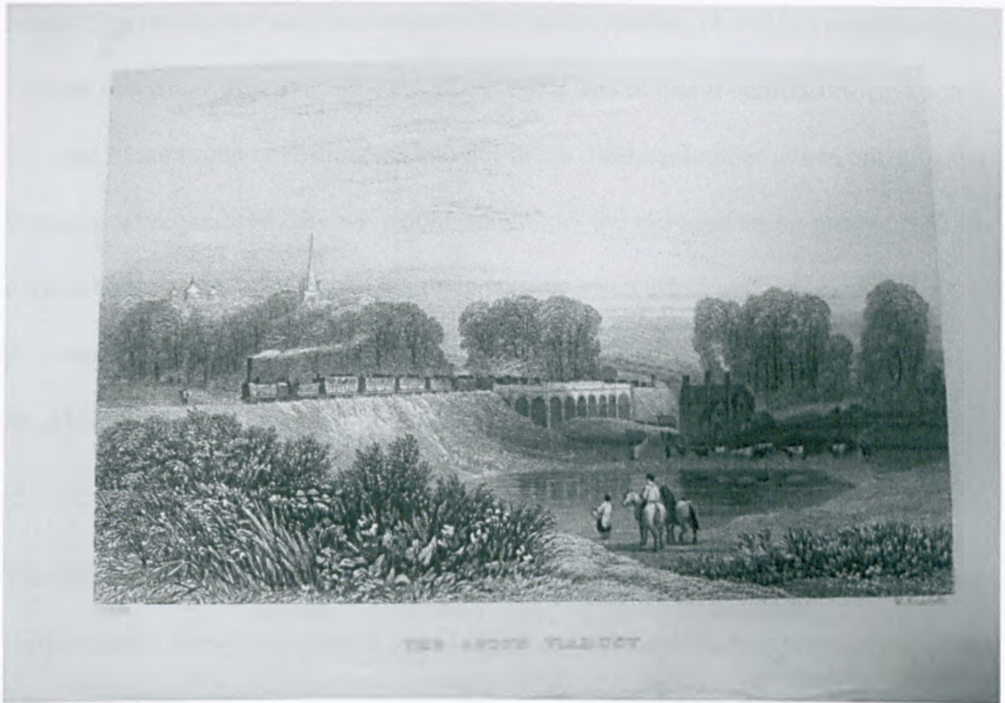
Figure 2.12. The Aston Viaduct , taken from Roscoe's Book of the Railway from Birmingham, Liverpool and Manchester (facing page 25).
