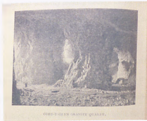
Figure 5.18. Coed-Y-Glyn Granite Quarry from North Wales.
