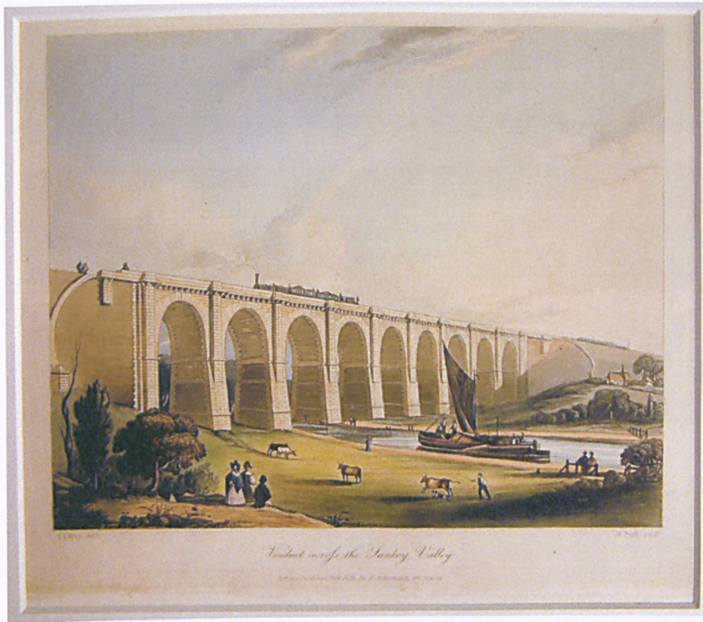
Figure 2.7. NRM 1975-8732. Viaduct Across the Sankey Valley.
