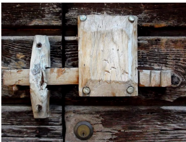
Figures 2.16, 2.17 Wooden lock from San Bernadetto, Italy showing lock housing (left) and keyhole (right) Soldati, 2012
