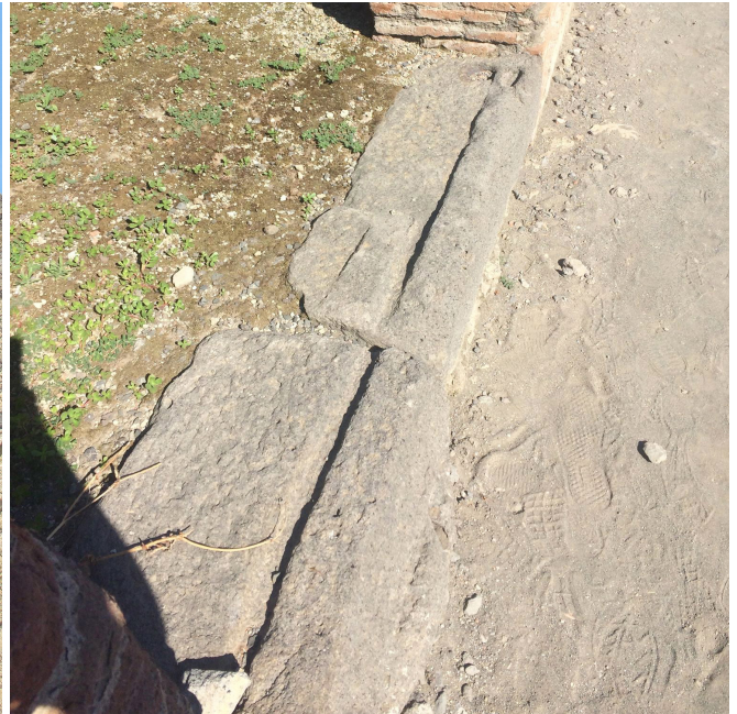
Figure 2.11 Shop threshold in Pompeii, grooved to lock shutters in place. Author's photograph (2015)
