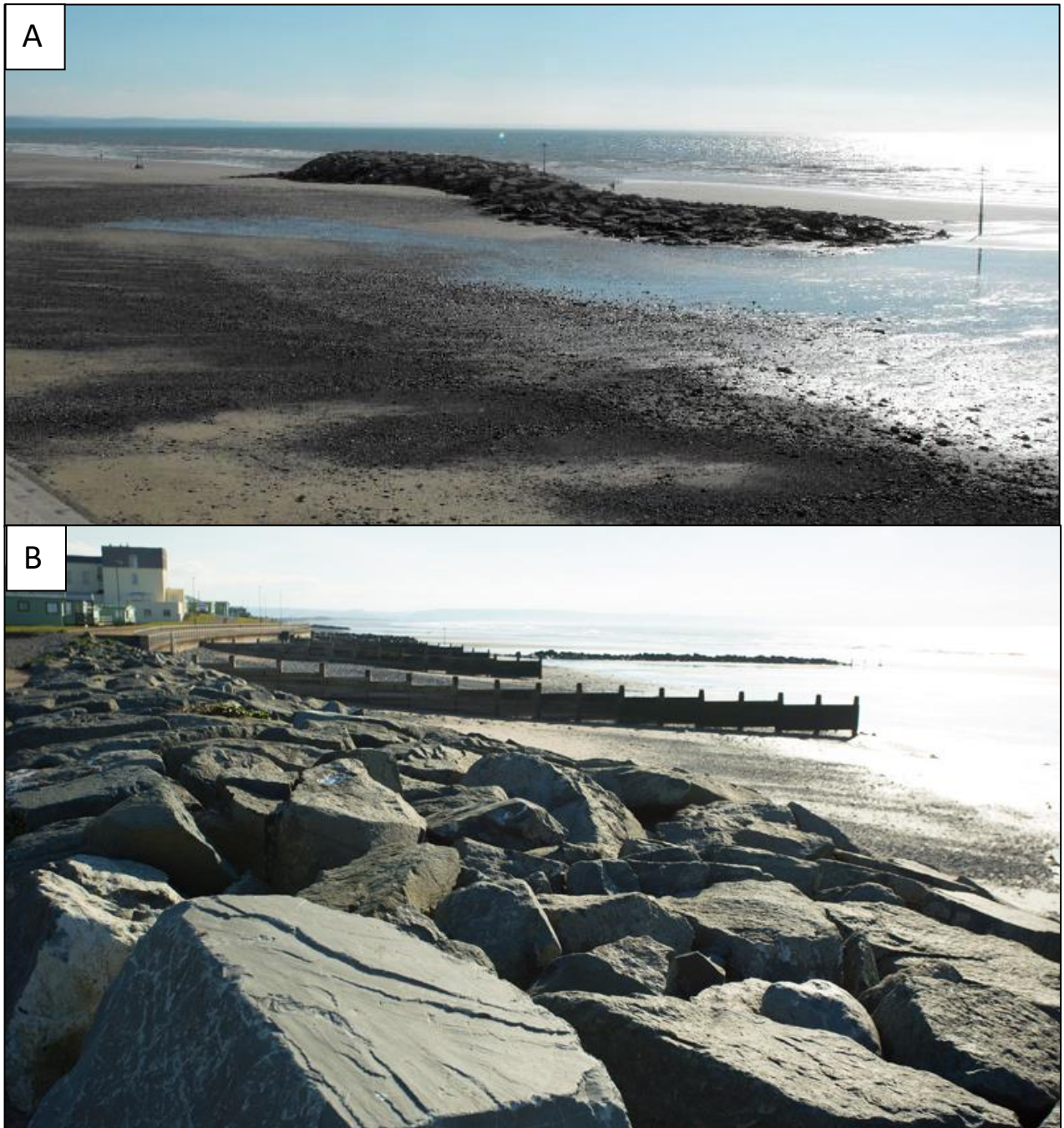
Figure 8.3. New defences built at Tywyn, including a detached breakwater (A) and a rock revetment (B). Photographs Copyright Penny Mayes
