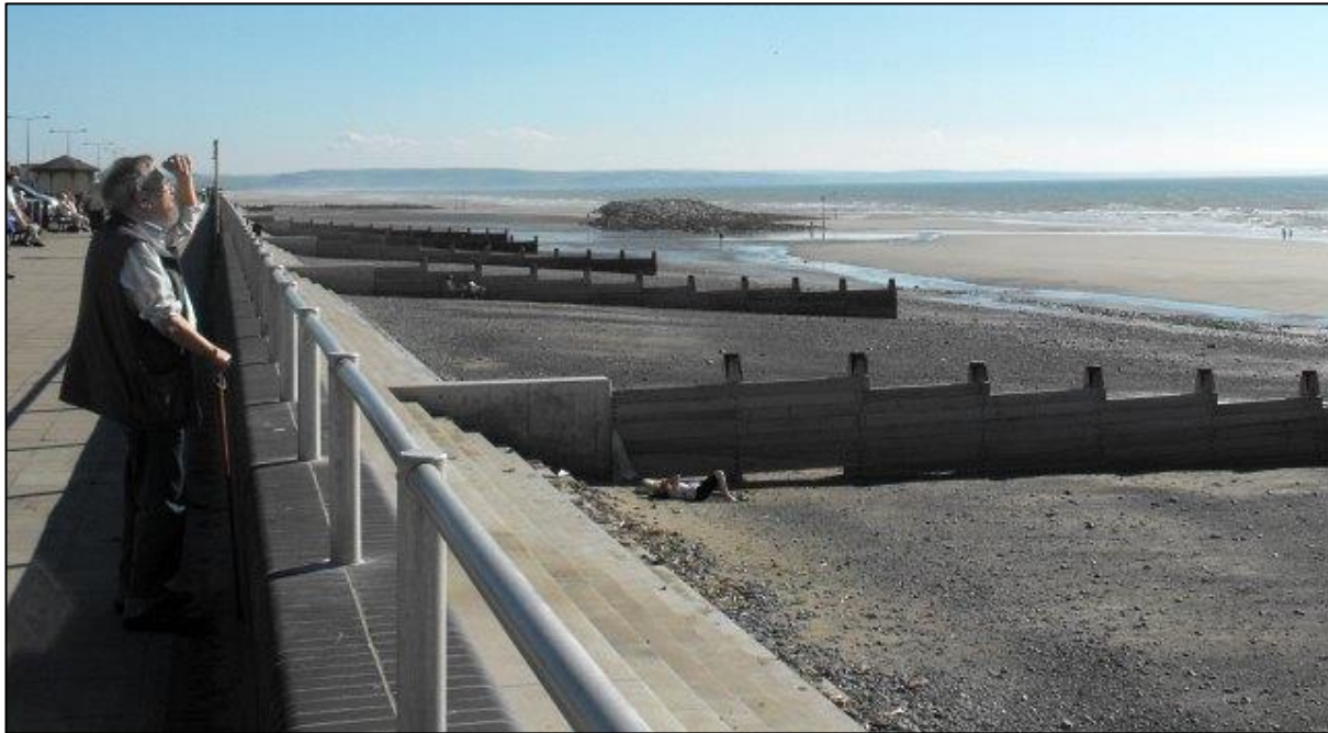
Figure 8.1. Late-20 th century sea wall built along the Tywyn frontage to protect the Victorian promenade. Present defences visible now also include wooden groynes. Photograph Copyright Penny Mayes
