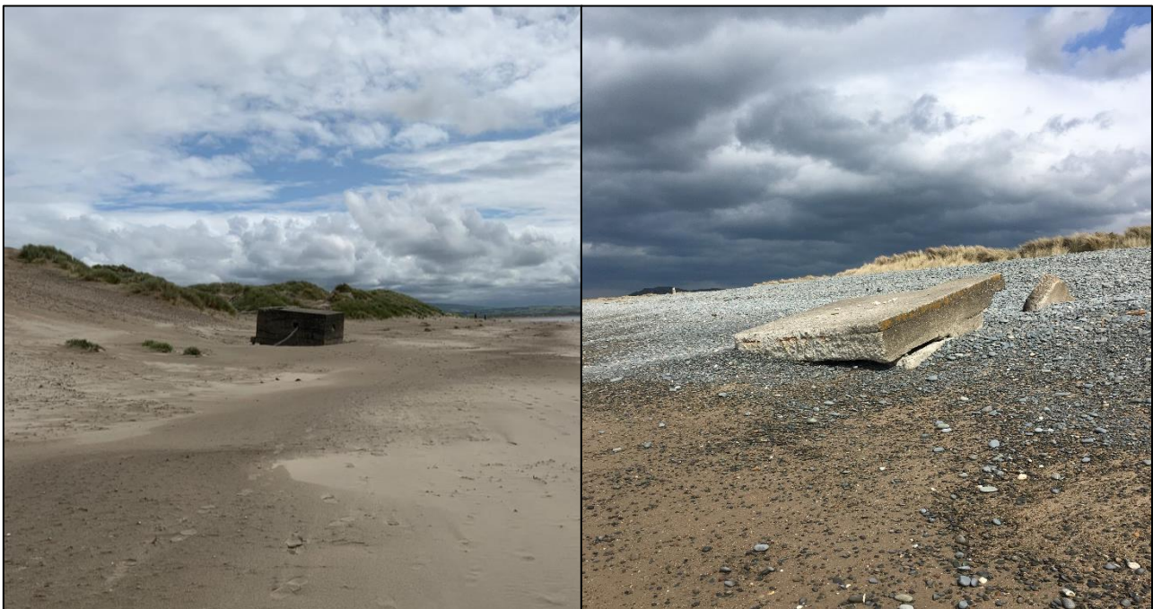
Figure 4.7. Two of the line of Second World War pillboxes between Tywyn and Aberdyfi
