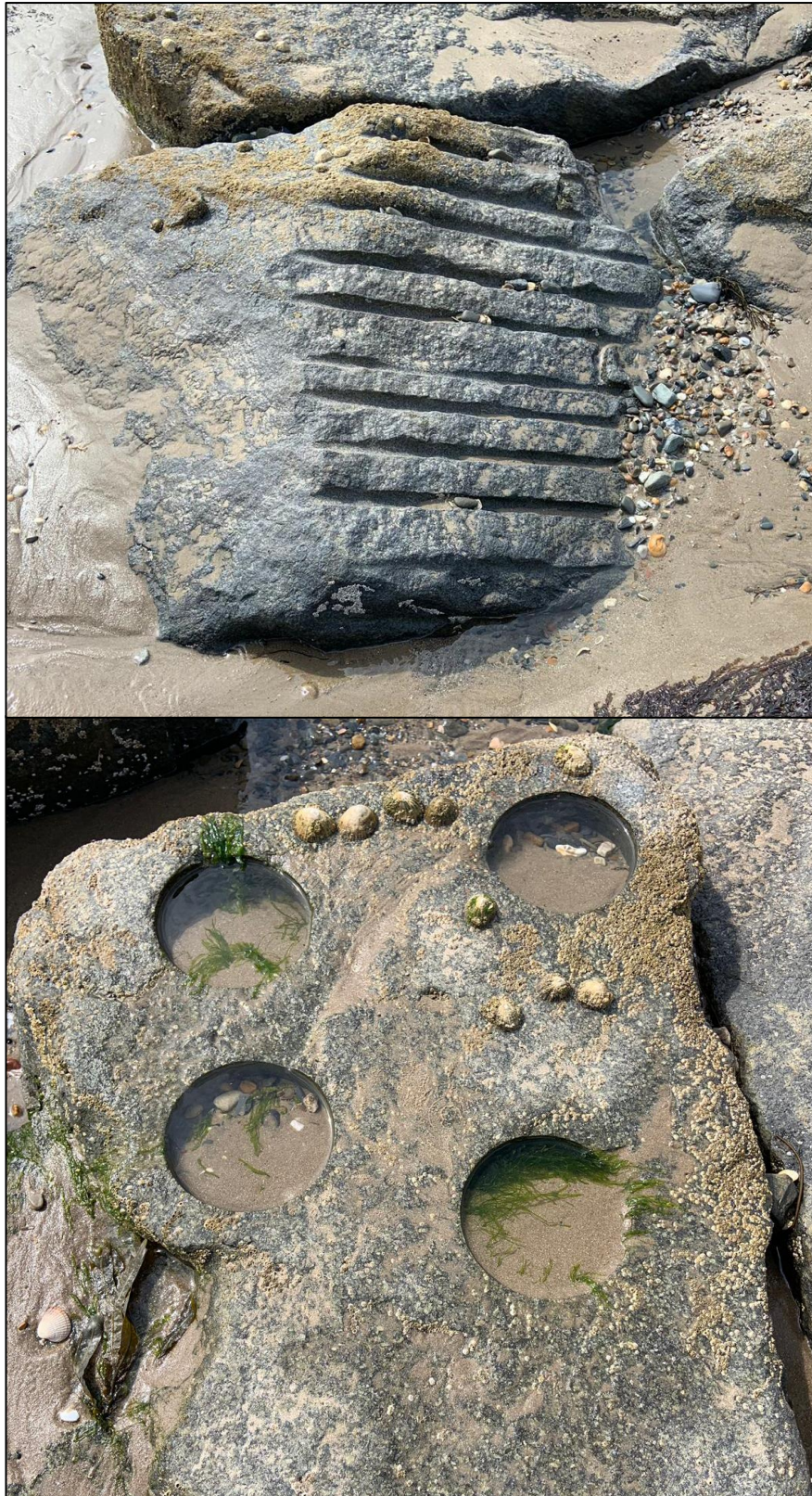
Figure 8.4. Evidence of ecological engineering features retroactively installed onto Tywyn breakwater by Evans et al. (2015).
