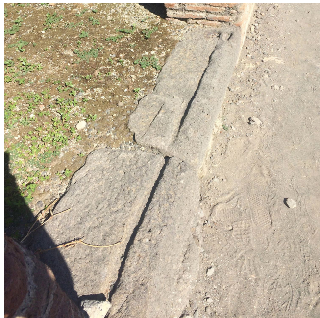
Figure 2.11 Shop threshold in Pompeii, grooved to lock shutters in place. Author's photograph (2015)
