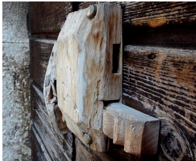
Figures 2.16, 2.17 Wooden lock from San Bernadetto, Italy showing lock housing (left) and keyhole (right) Soldati, 2012
