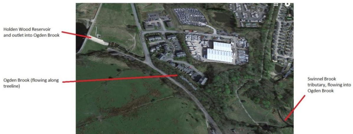
Figure 4.2: Satellite view of Holden Wood Reservoir and Ogden Brook
