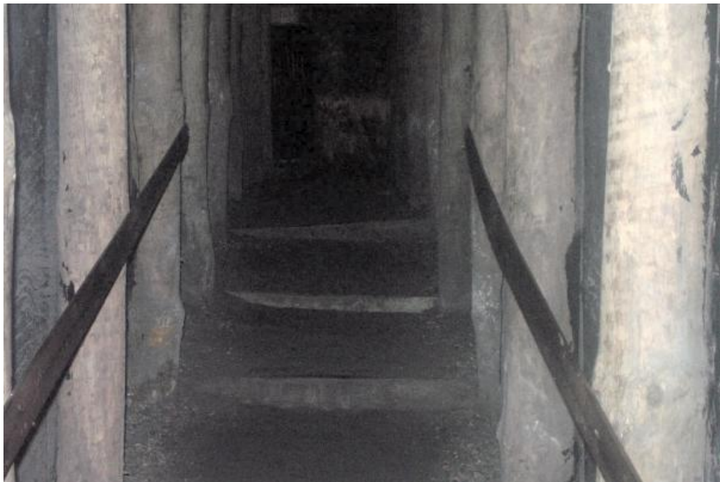
Figure 31. Underground 'Roadway', NCMME
