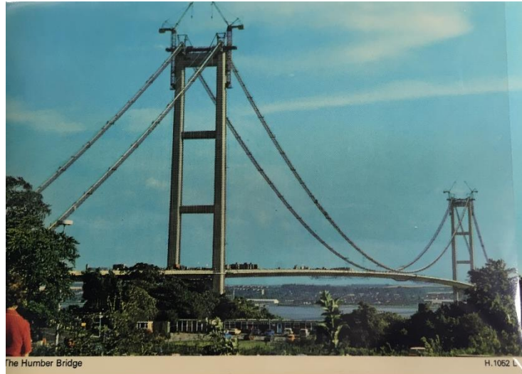
Image 14: a postcard (undated, unwritten) depicting the Humber Bridge under construction, kept by Larkin within one of his photograph albums. 88
