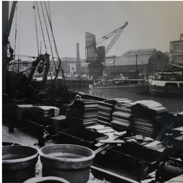
Image 16: photograph from the poet's collection, of cranes and machinery at Hull Docks, taken during the filming of the BBC 'Monitor' programme (1964). 106
