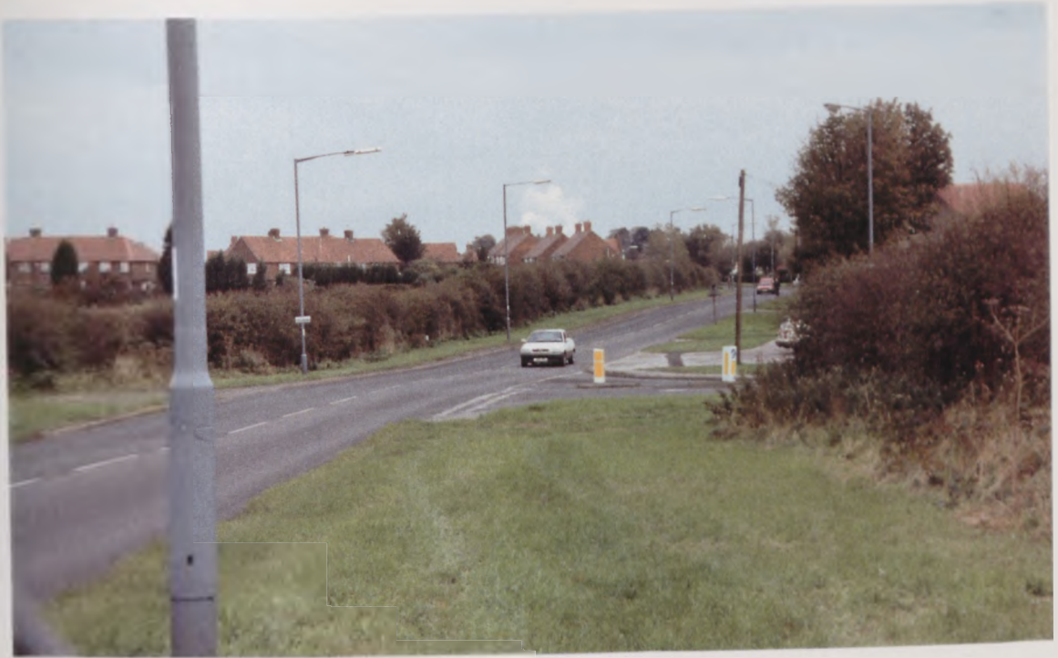
Figure A.5: Askham Lane - before situation
