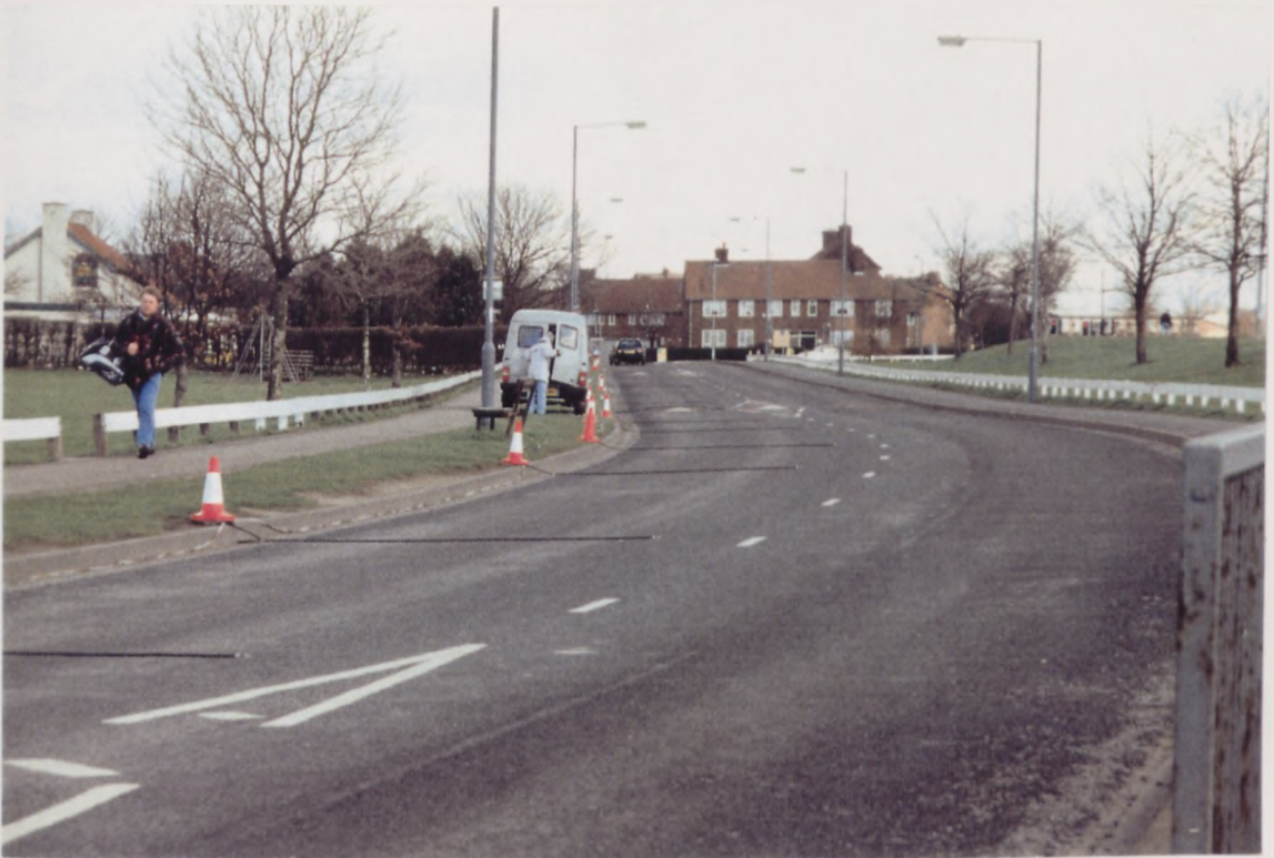
Figure 4.8: Experiment Conducted at Foxwood Lane East (towards Gale Lane)
