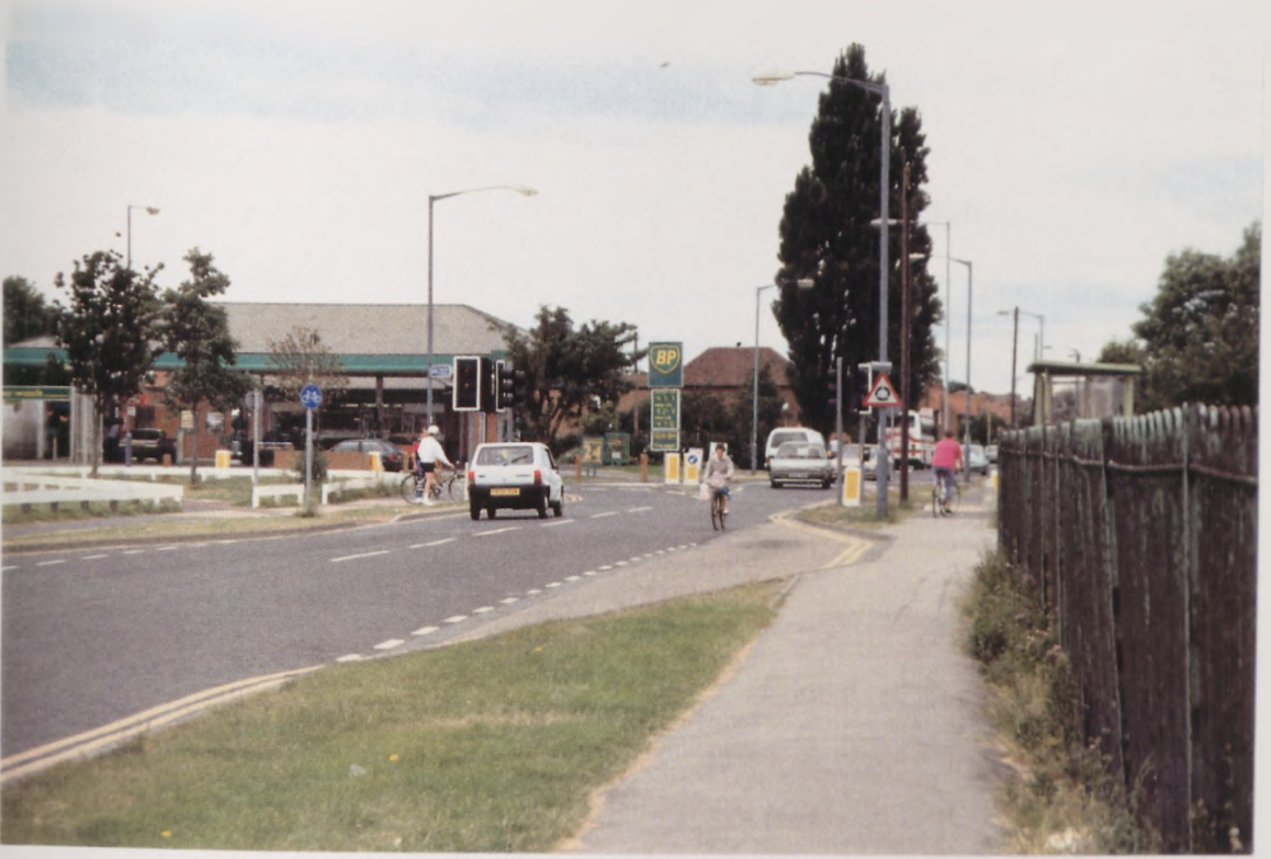
Figure A.1: Thanet Road towards Gale Lane and Foxwood Lane (on the left)
