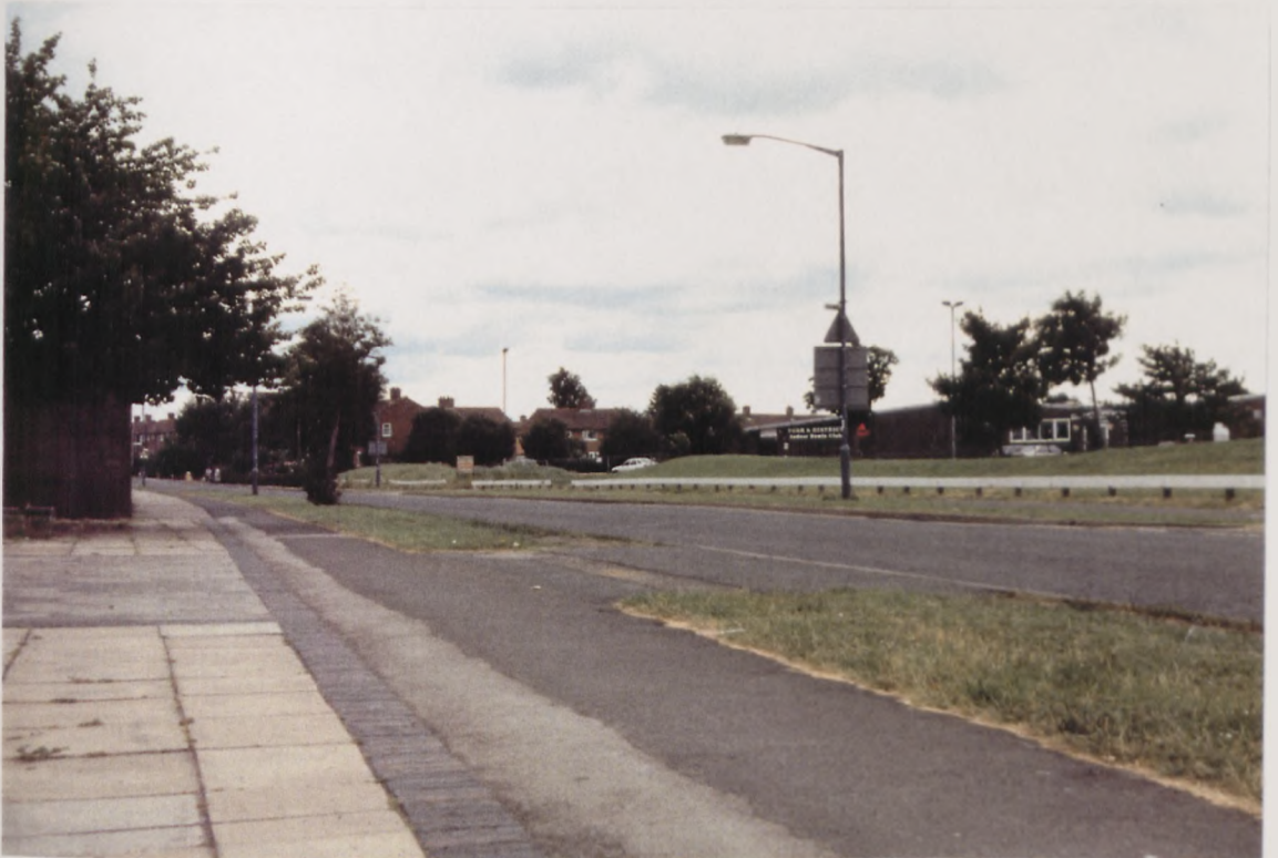
Figure A.2: Thanet Road Station - measurement point
