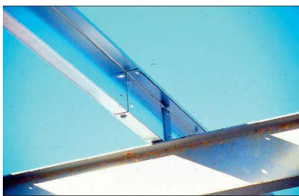
Fig. 2.19. Continuous lapped Z-purlin configuration (Pham et al., 2014)
