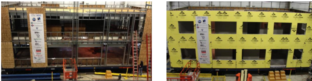
Fig. 2.21. A full-scale shake table test on a CFS framed building (Nakata et al., 2012, Schafer et al., 2016)
