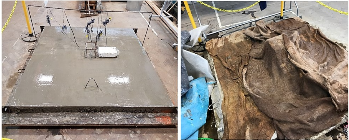
Figure 3-12. Slab specimen being poured and cured
