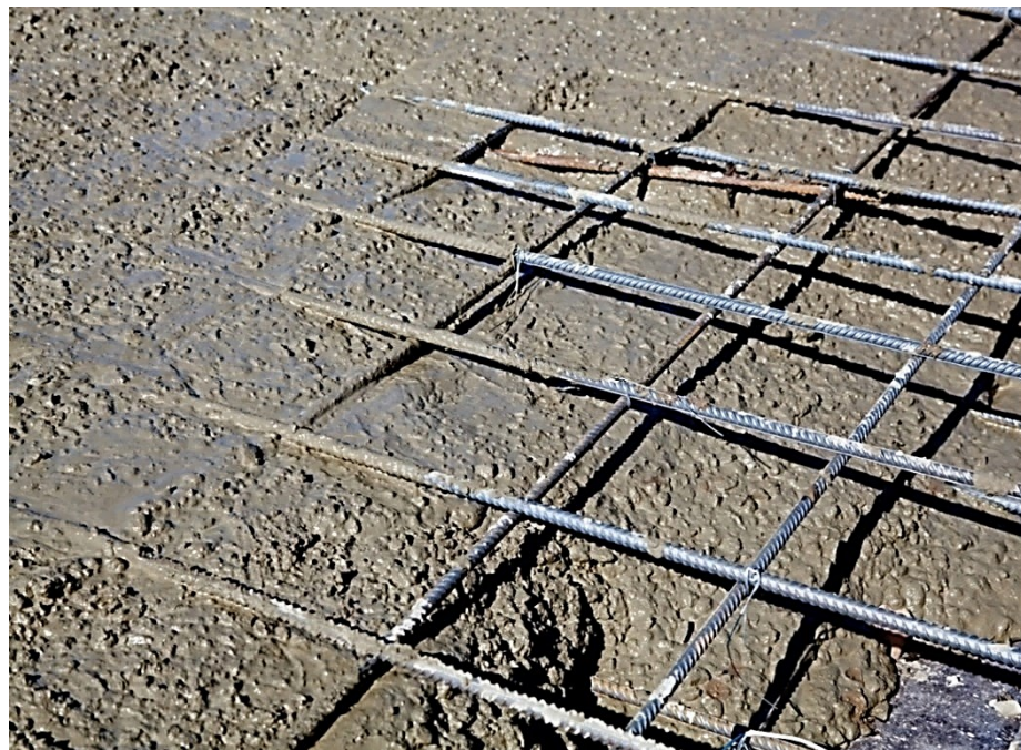
Figure 2-34. Reinforcement inside poured fresh concrete
