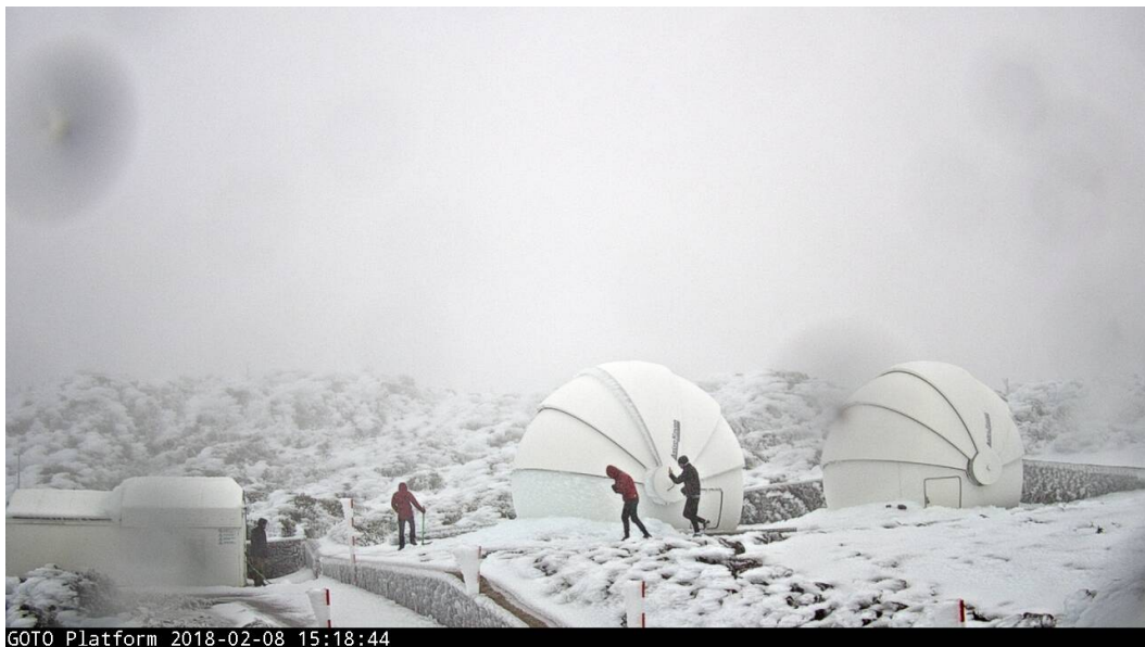
Figure 8.21: External webcam image showing the ice rescue team. Note the build up of ice visible on the northern side of the upper shutter of the (empty) left-hand dome. A similar build up caused the upper shutter on the right-hand dome containing GOTO to be pulled open.
