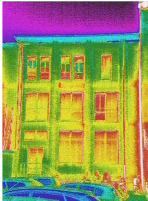
Figure 1.3. Example thermographic image of building façade [20]
