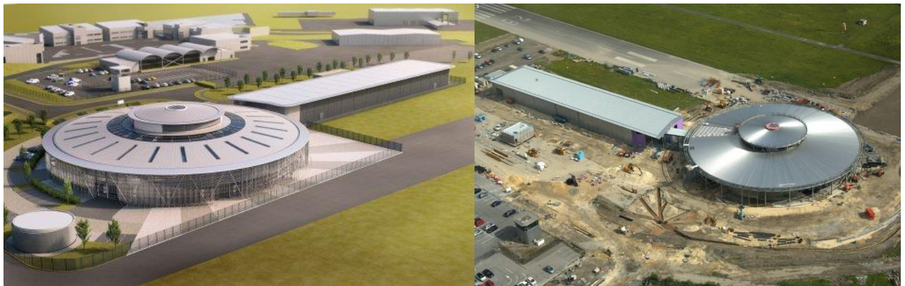
Figure 3.5. (left) Artistic render of F2050 [137], (right) Aerial View of F2050 under construction [138]
