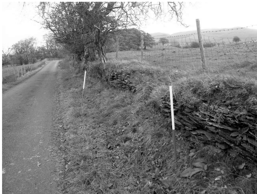
Figure 37: Bank supported by slate fragments on the road to Sosgill.
