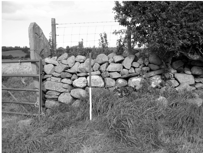
Figure 31: A wall constructed using water worn stones near Mosser Moss.
