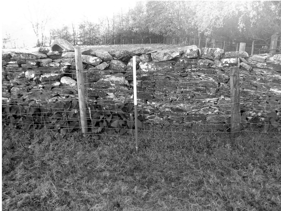
Figure 28: A wall with jumble capping near to Bramley Farm
