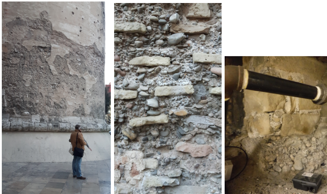
Hot mixed, rammed concrete, Valencia town wall.
