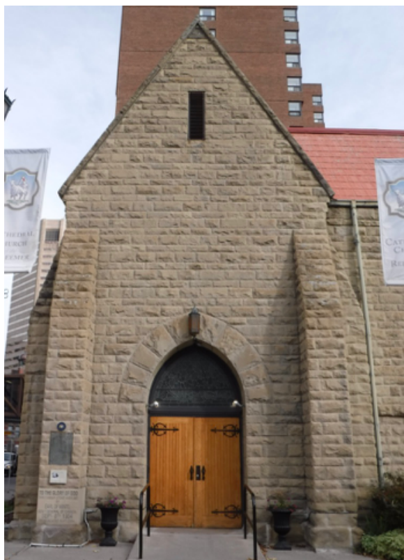
Figure 16 Cathedral of St Luke the Redeemer, 1905-06, Calgary, Alberta (see Appendix Eleven No.10). Hot mixed lime mortar with small volumes of Portland cement added.
