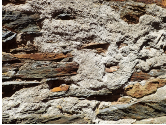
Figures 64 & 65 Asturias, Spain; clay mortar, hot mixed lime renders.
