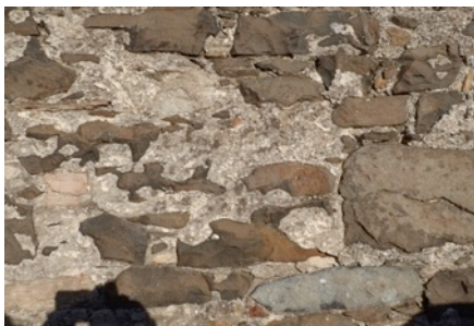
Figure 24: hot mixed half-harling, Lindisfarne; Figure 25: hot mixed and placed internal plasters, ironstone workers houses, Rosedale, North Yorkshire (see Appendix Eleven No.11)
