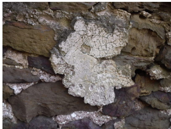
Figure 24: hot mixed half-harling, Lindisfarne; Figure 25: hot mixed and placed internal plasters, ironstone workers houses, Rosedale, North Yorkshire (see Appendix Eleven No.11)
