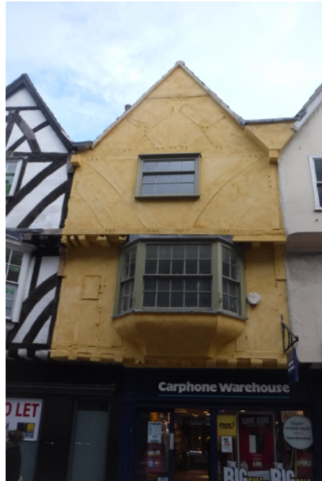
Figure 98 hot limewash to interior of York House, Malton, 2010. Figure 99 Hot limewash to 20 Coney Street, York, 2018.
