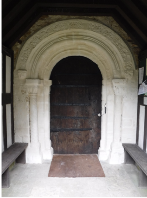
Figure 96: Hot mixed aggregated limewash (sheltercoat) Crowland Abbey 2016. Figure 97: Hot limewash, All Saints, Foston, North Yorkshire 2018
