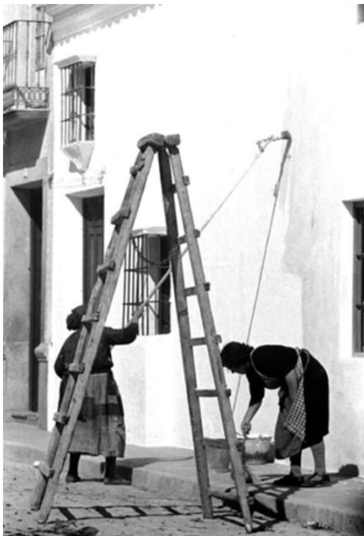
Figure 93 Routine limewashing in Spain, earlier 20thC (Museo de Cal de Moron)
