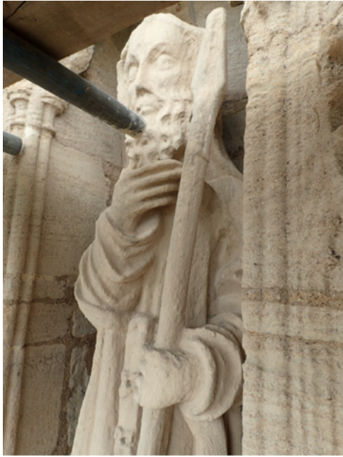
Figure 96: Hot mixed aggregated limewash (sheltercoat) Crowland Abbey 2016. Figure 97: Hot limewash, All Saints, Foston, North Yorkshire 2018
