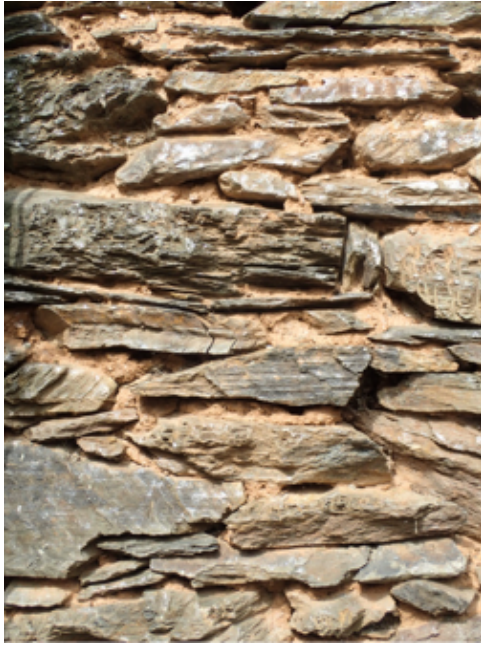
Figures 64 & 65 Asturias, Spain; clay mortar, hot mixed lime renders.
