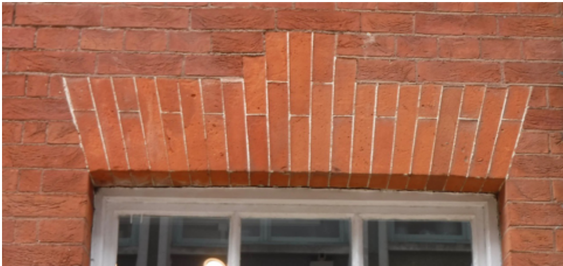
Figure 48: gauged brickwork, York.
