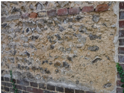
Figure 80 Flint laid in earth-lime mortar. Calvados, Normandy.
