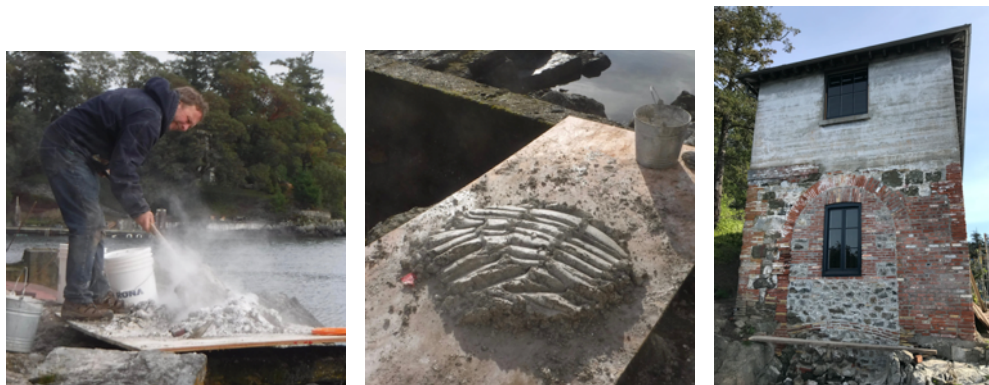
Figures 51-54: the ordinary method . Figure 55: the mortar in place
