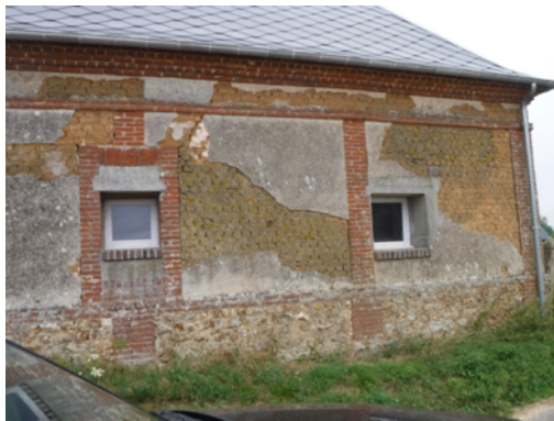
Figure 81 Adobe construction, Calvados
