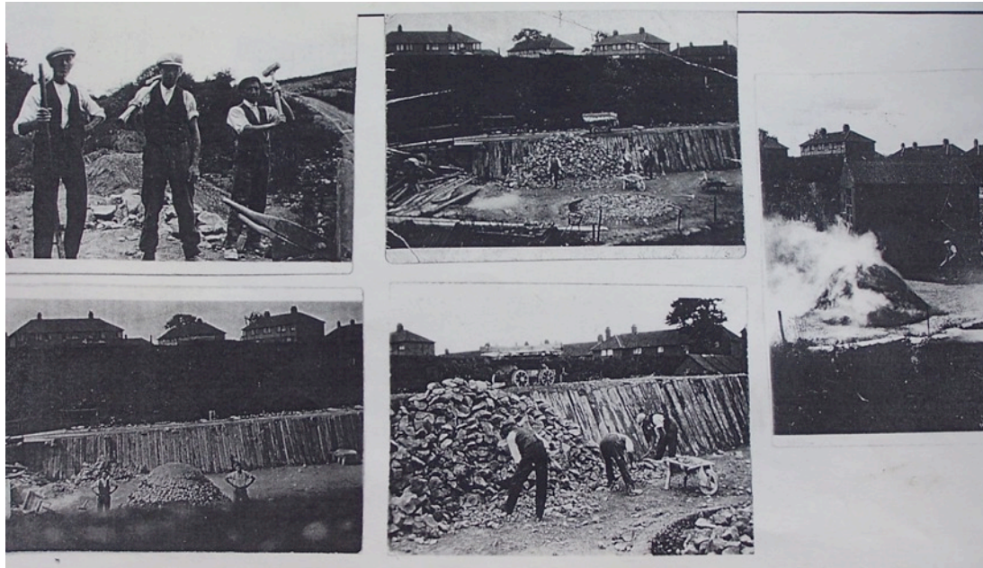
Figure 2 Lime-burning at its most simple, Malton, 1930s. This was used in the construction of social housing, some of it visible in the background. (Image: Eric Blades).
