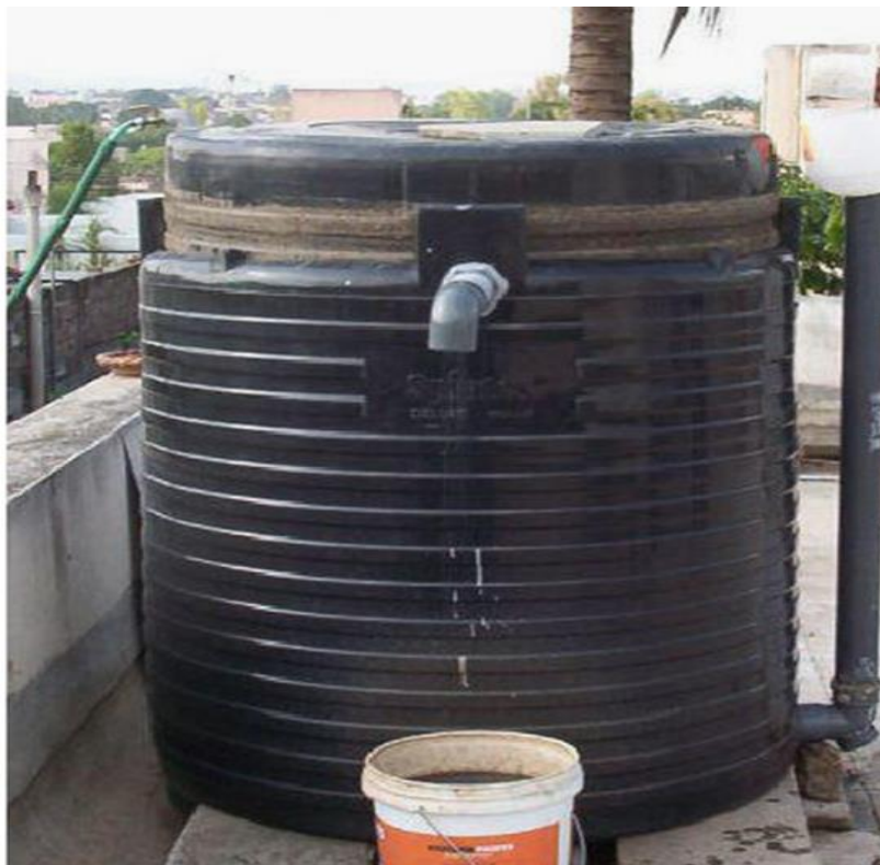
Figure 2.9 floating drum design made from HDPE material [190].
