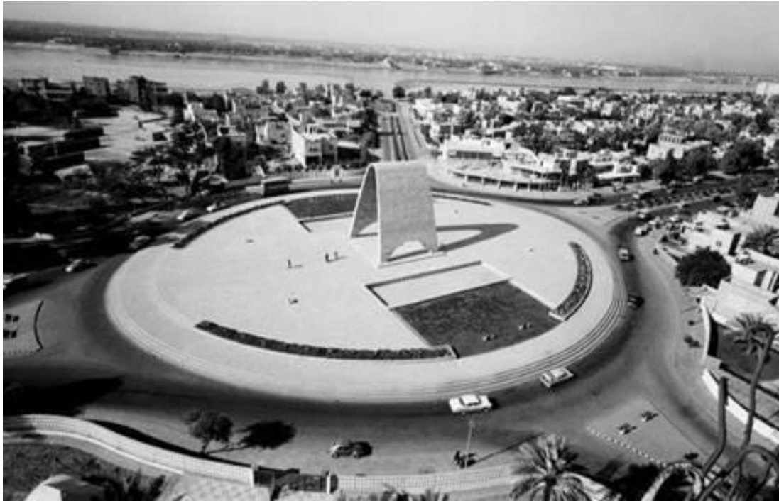
Figure 3-19: Monument for the Unknown Soldier in Baghdad in 1960 in Firdos Square. Designed by Rifat Chadirji, it was a modern adaption of the arch of Ctesiphon which could consider as one of the oldest feature In the Iraqi architecture
