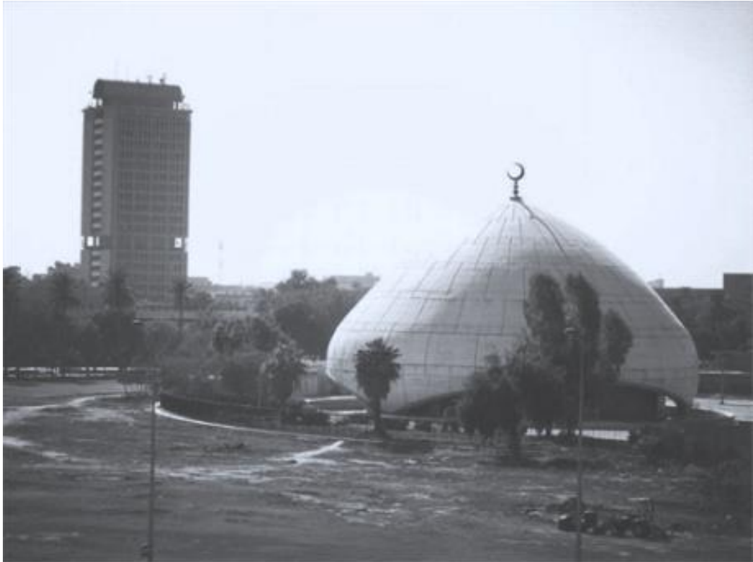
Figure 7-21 : View of the university's faculty tower and the university's mosque with its large dome that supported by three main points which suspended over the water lake.
