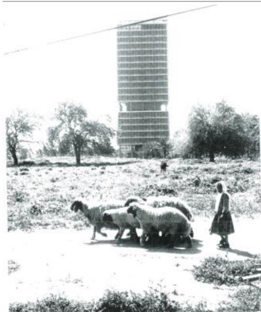
Figure 7-29: The University Campus location, and the Faculty Tower, during the time when the construction stopped. And the land has been used by farmers
