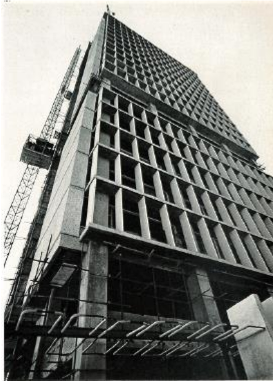
Figure 7-17: The faculty tower, during its construction.
