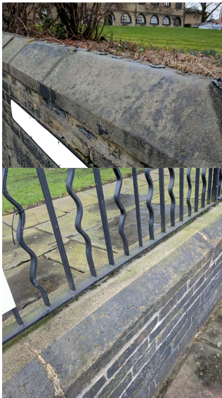
Figure 4f: Repairs to a boundary wall, which Firm17SM felt could have conserved the 'rounded head' (Top: before; Bottom: after)
