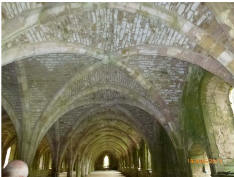
Figure 3n: Consolidating the cellarium vaults was standard winter work for fully trained masons
