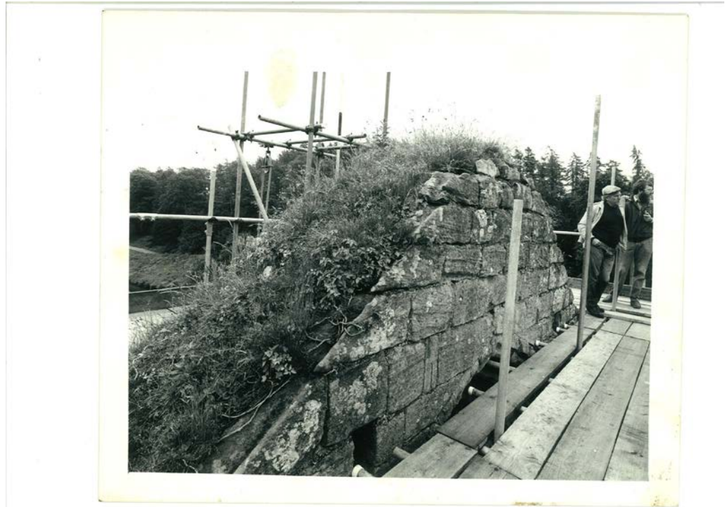
Figure 3k: Dave Sweeney on the scaffold at Fountains
