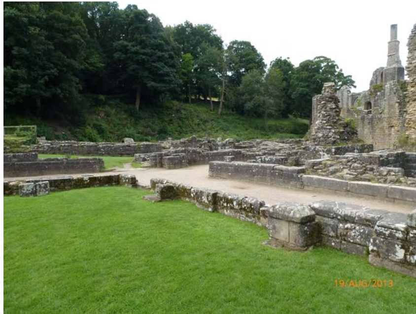
Figure 3j: The low-lying walls of the infirmary were among the first worked on by MPBW masons
