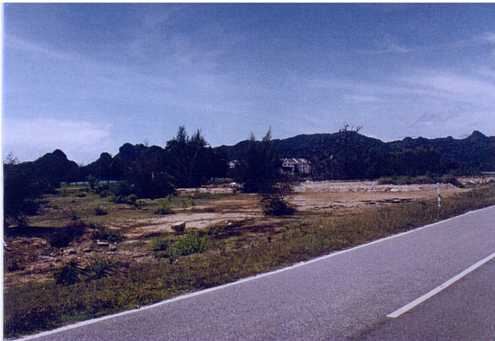
Fig.6-4 Part of the site that has been abandoned.
