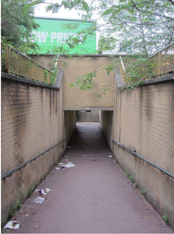
Figure 17 Pedestrian walkway and road bridge at Dudley Hill
