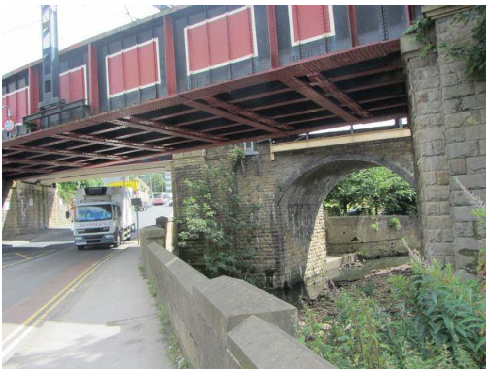
Figure 18 Bridge crossings at Shipley
