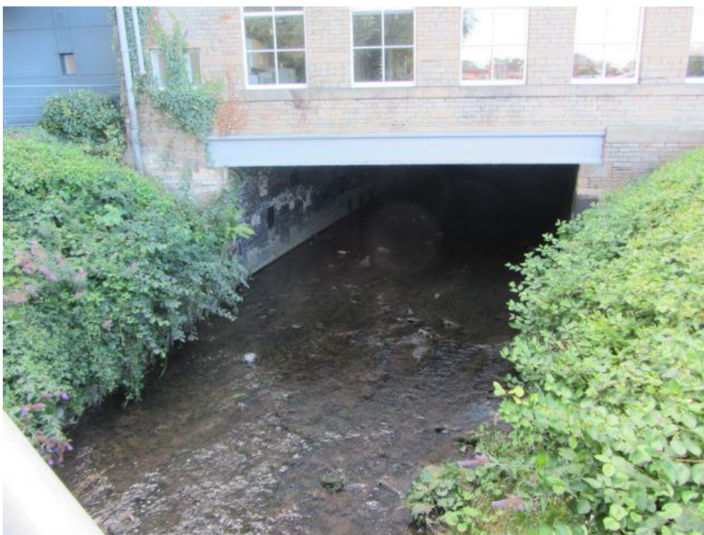
Figure 15 The beck emerges from underneath a renovated mill
