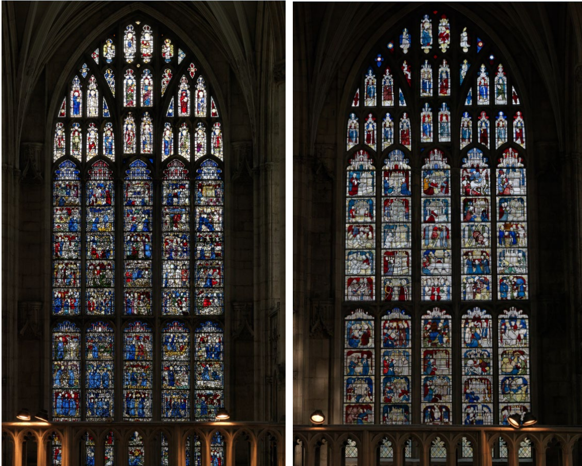
Figure 4.4. The use of the same stonework design in (left) the St Cuthbert Window (s7), top half, c.1440, and (right) the St William Window (n7), top half, c.1414 (Images YGT © DCYM)
