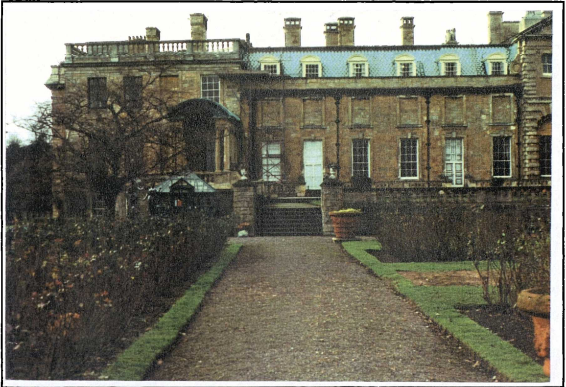
Figure 134 The Welbeck Garden. East Terraces looking towards the Abbey. Alley adorned with Italian vases.
