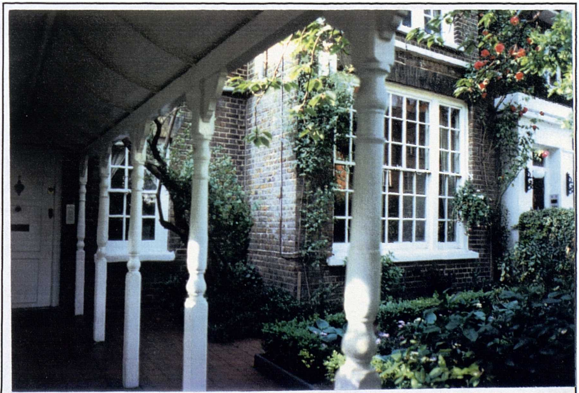
Figure 44 54 Bedford Gardens. Detail: Front Entrance.
