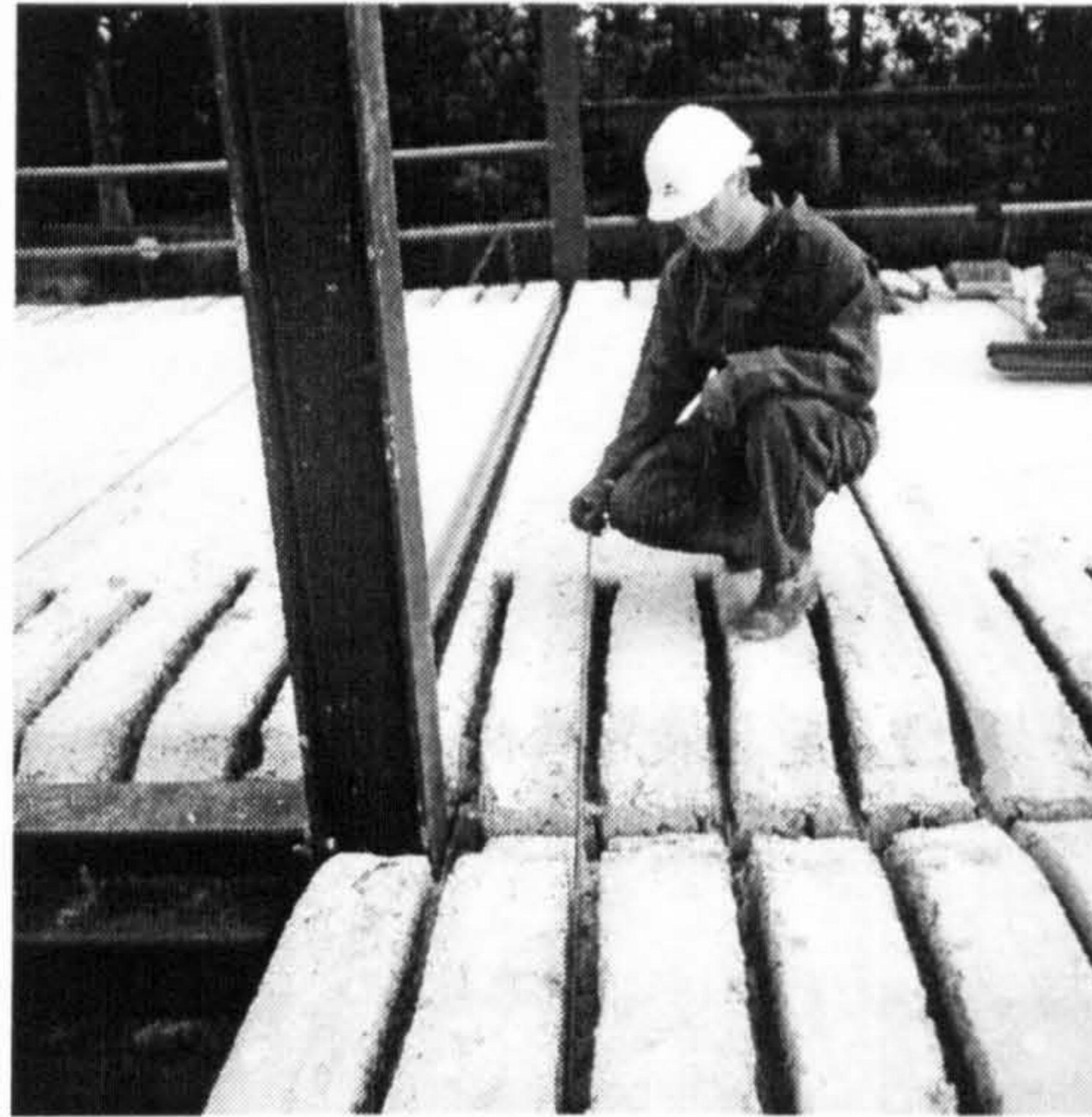
Figure 2.2 Composite beam with tapered-end hollow core slabs during construction
