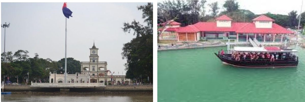
Figure 3.9: New development buildings in Tanjung Emas Promenade within the royal precinct
