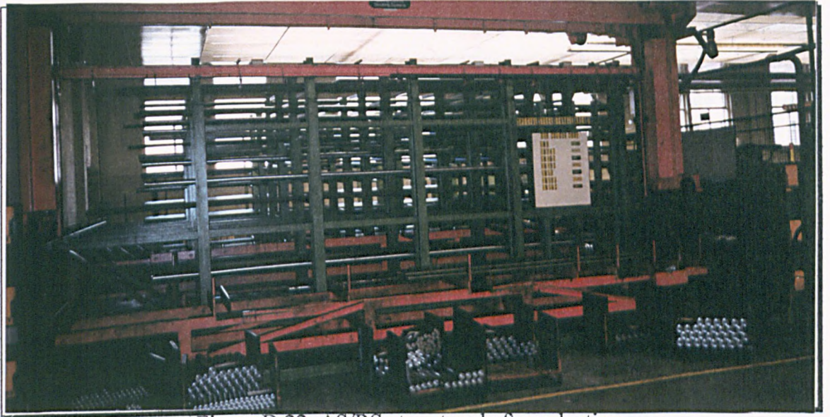
Figure D.22. AS/RS at motor shaft production.
