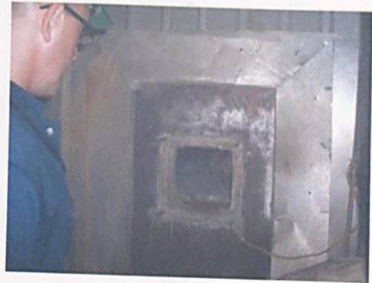
Figure 4.8 An opening hole after the viewing port was removed.
