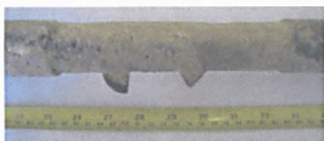
Figure 3 Coated coupons – wall section
