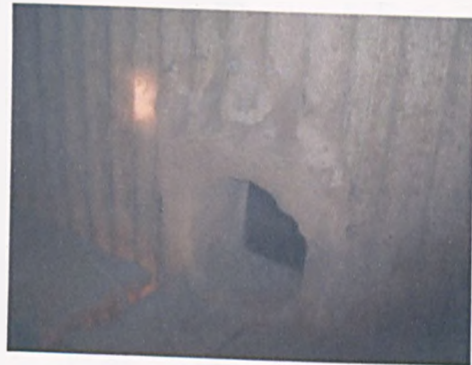
Figure 4.10 Inner side of the wall at the location of probe No.1
