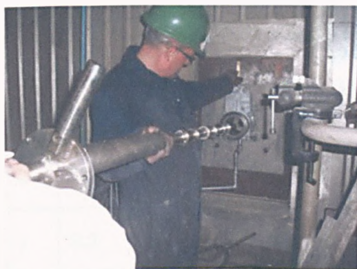
Figure 4.14 Installation of the sampling probe No.1
