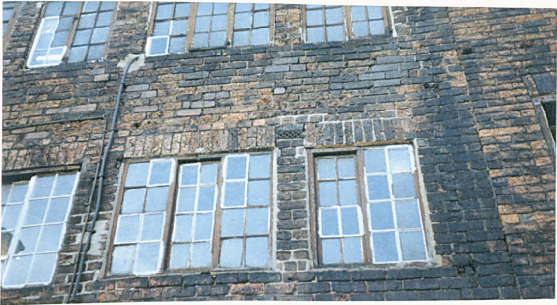
Figure 28a: Traditional cutlery workshop windows with a horizontal slide opening.
