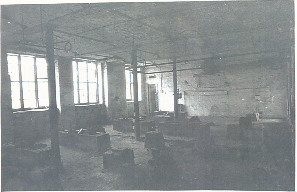
Figure 13a: Cast iron columns, Butcher's Wheel
