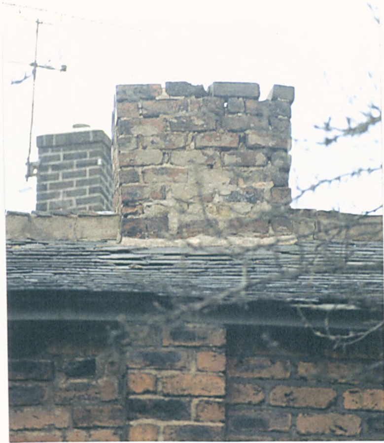
Figure 17a: Hearth Chimney, Cross Hill, Ecclesfield. File cutter's workshop.
