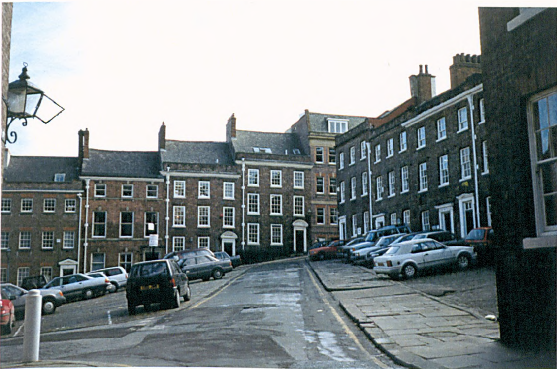
Figure 36c: Many of the windows found on office blocks and packing shops of the large and medium scale works resemble those found on Georgian town houses such as those in Paradise Square.
