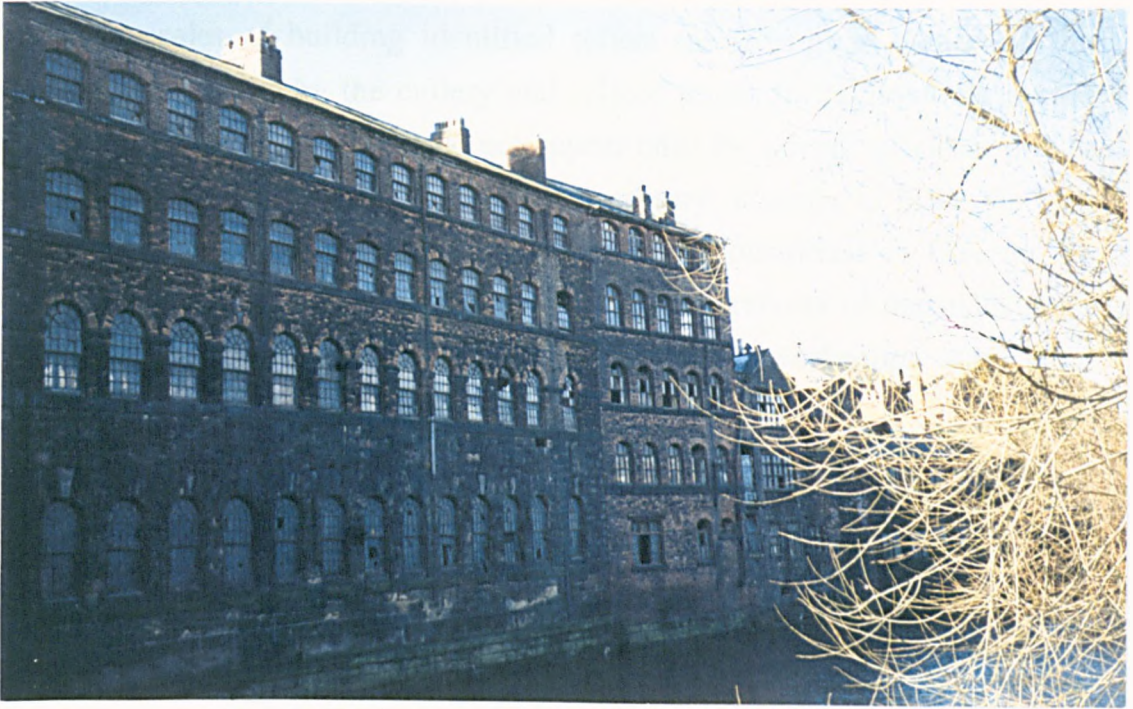
Figure 5b: Cornish Place. The workshop range facing the river is five storeys.
