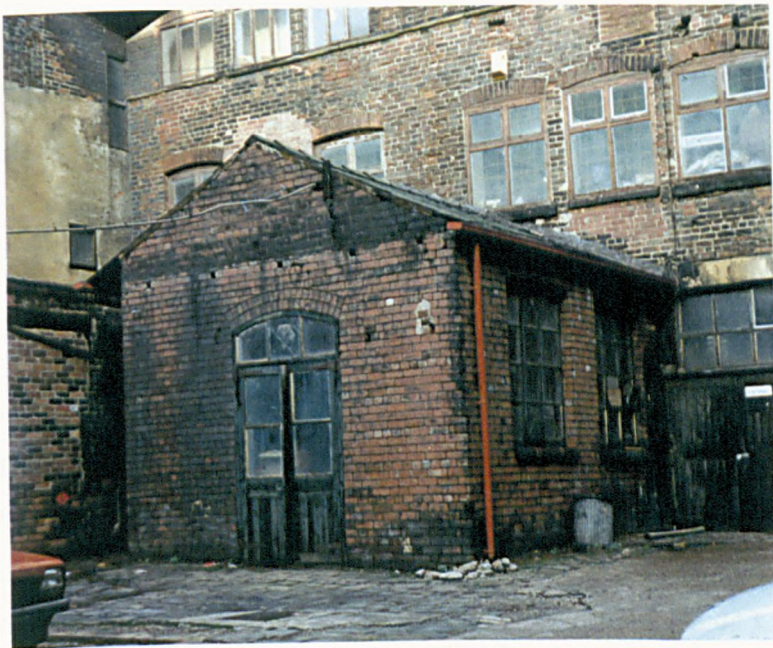
Figure 39: Generating room at Butcher's Wheel built between 1905 and 1923 (A1)
