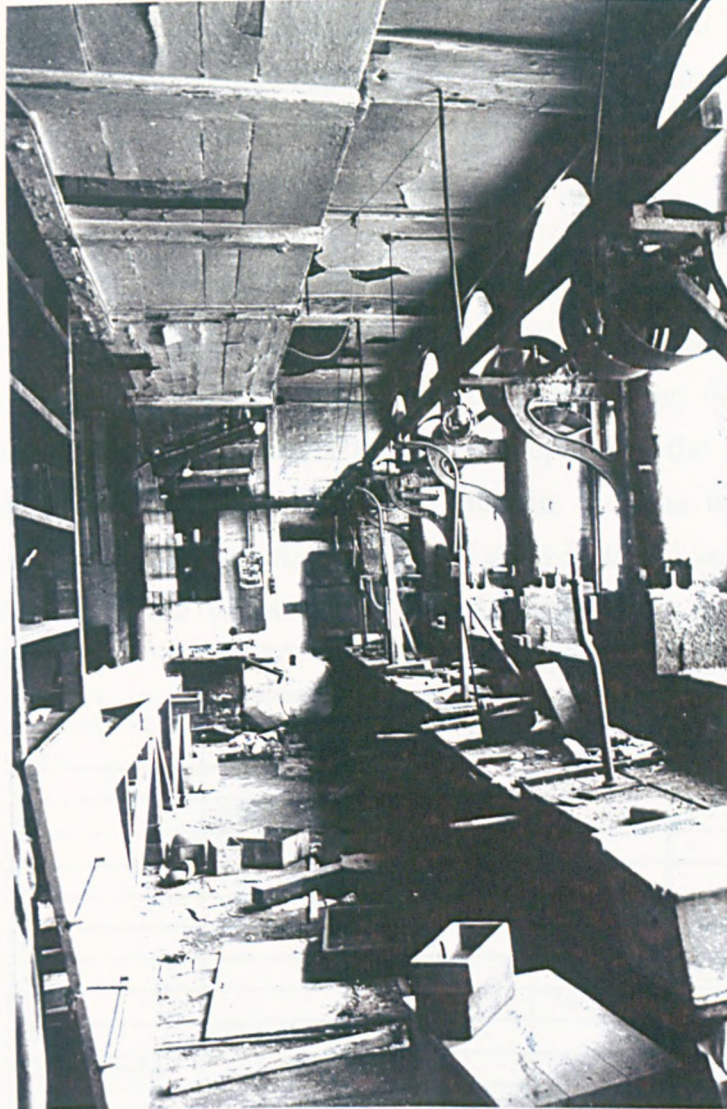
Figure 35: Wall brackets for line shafting at Cornish Place
