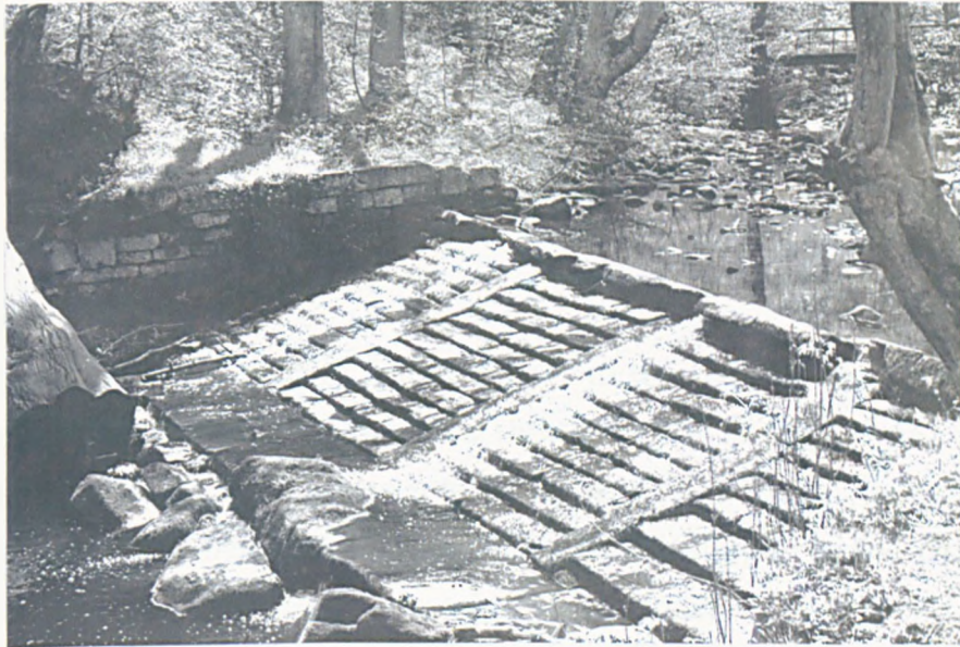
Figure 4: Example of weirs constructed in bays on the Rivelin. Above Wolf Wheel, below a weir built in the vernacular style at Mousehole Forge.
