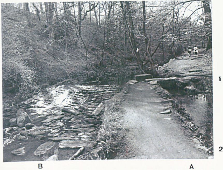
Figure 3: Example of a weir at Frank Wheel (Rivelin) where the top kerb remains but the bottom one has begun to erode with lack of maintenance. The head goit can be seen at A1 and note the height of the head race above the river (B2).
