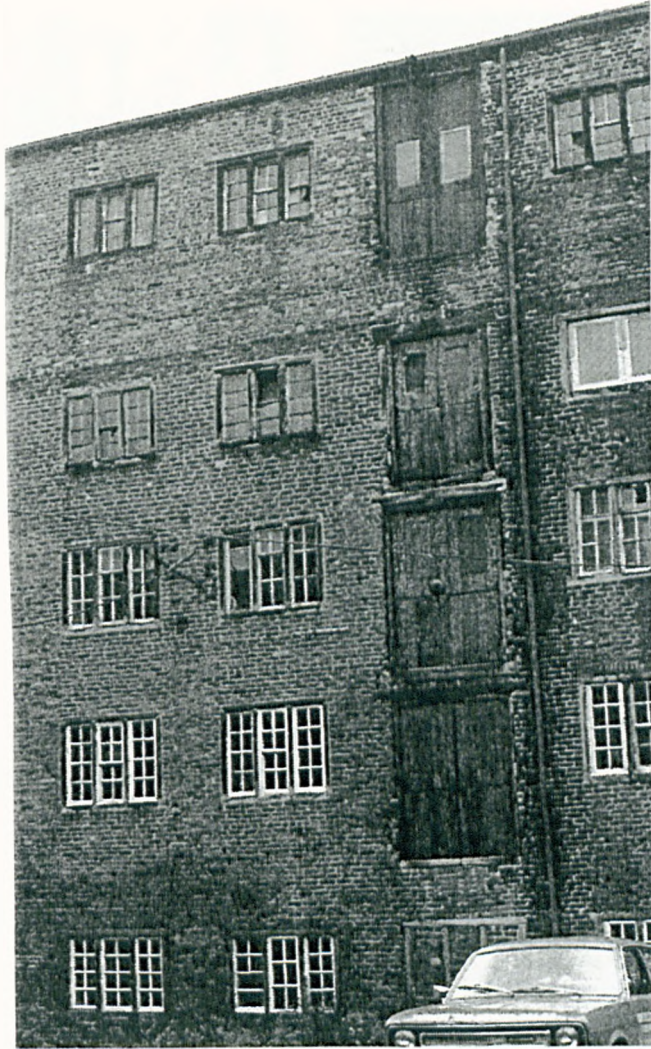
Figure 31: One of the few examples where the windows are almost identical to the fenestration found on most cutlery workshops. This is Carlton Mill, Sowerby Bridge. (From Jones E, 1985;32)
