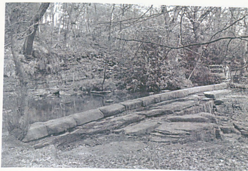
Figure 2: Third Coppice (Rivelin), the weir here is constructed from the natural bedrock. Note however that the kerb stones at the top of the weir are held together by iron staples.
