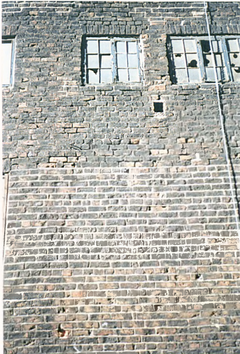
Figure 7b: Common Bond used in the construction of the workshop block at Kendal Works.
