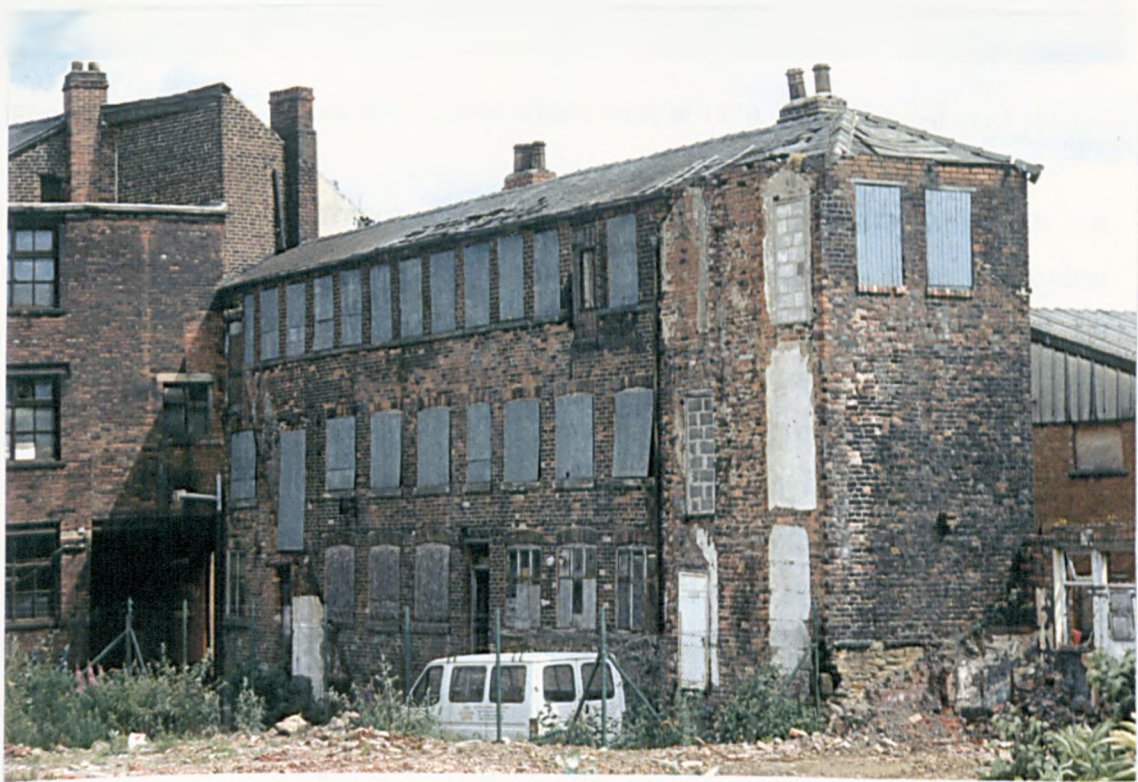
Figure 1a : The workshop block at Sylvester Works, dated c1840 was listed before 1995.
