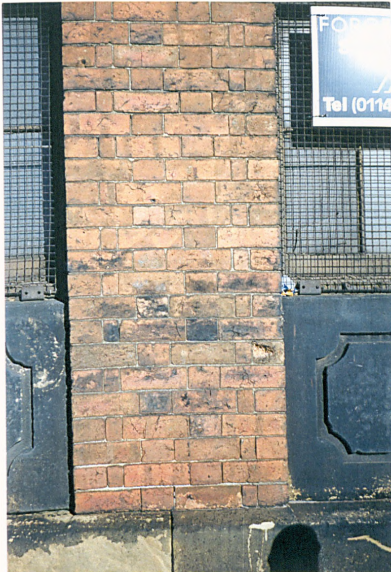
Figure 7f: Flemish Bond used in the construction of James Dixon's frontage block.
