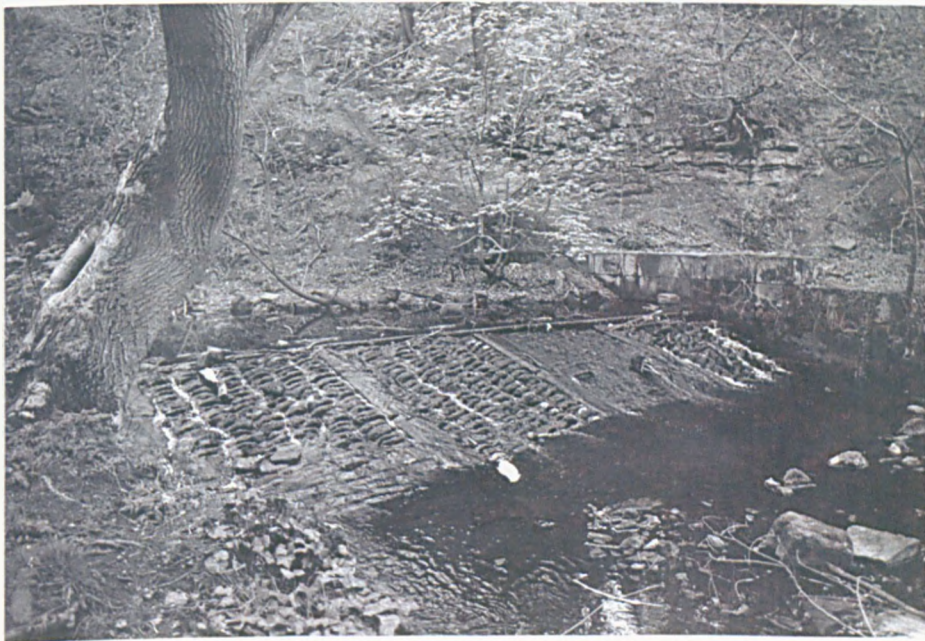
Figure 4: Example of weirs constructed in bays on the Rivelin. Above Wolf Wheel, below a weir built in the vernacular style at Mousehole Forge.
