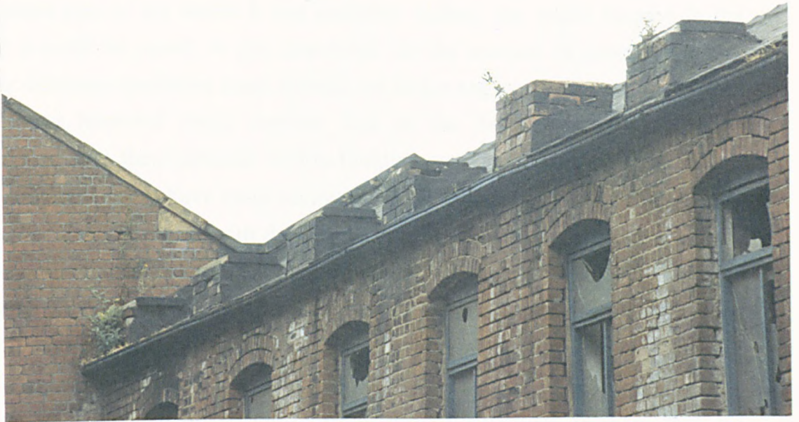
Figure 19: Hearth Chimneys, Alfred Beckett's, Ball Street.
