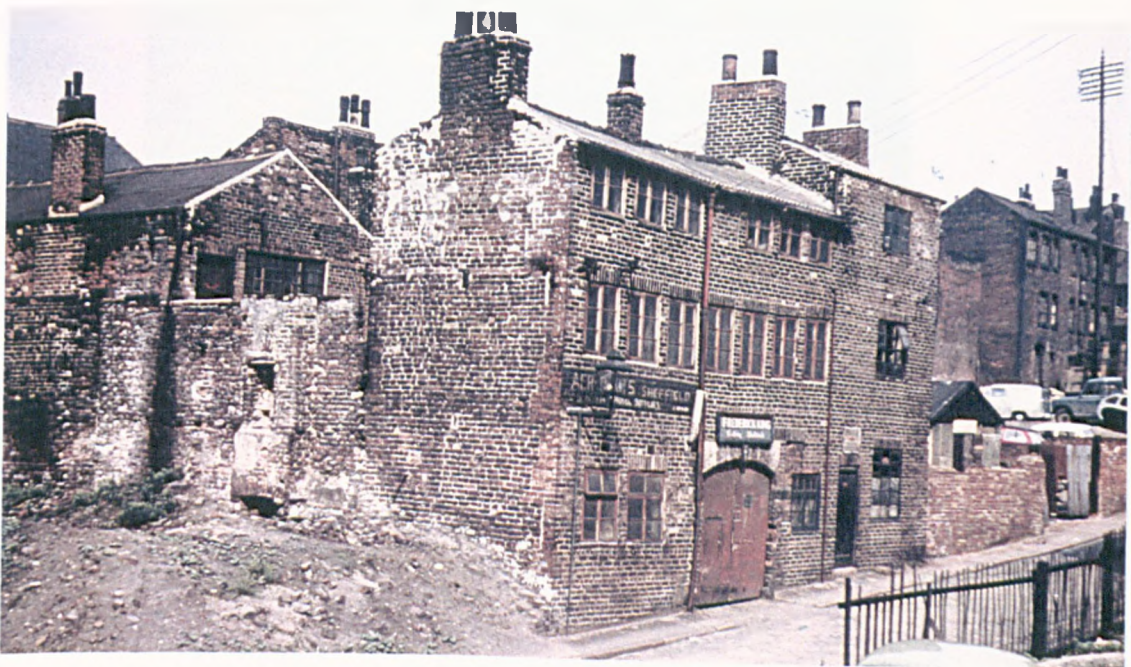
Figure 29: Typical Windows are usually found on the top storeys of buildings as at these workshops Rockingham Lane (JW Sibley Collection, Local Studies Library;1961)
