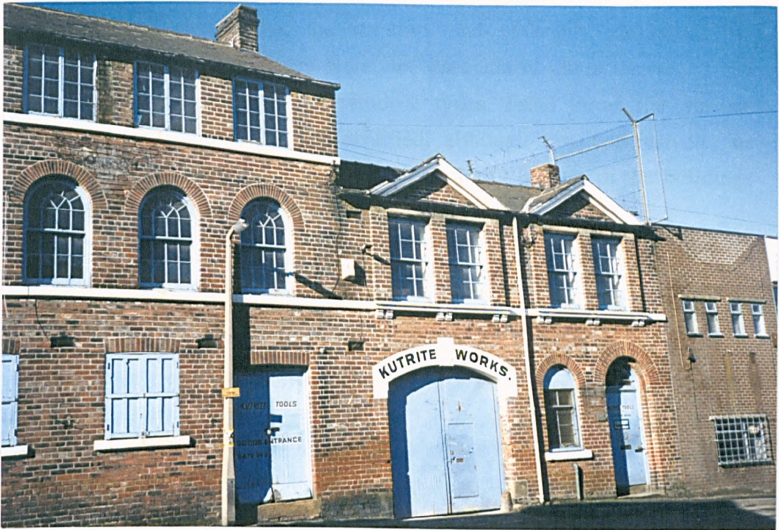
Figure 36b: Kutrite Works, Smithfield. Note the round headed windows probably indicating a showroom, office or warehouse and the typical workshop windows above.
