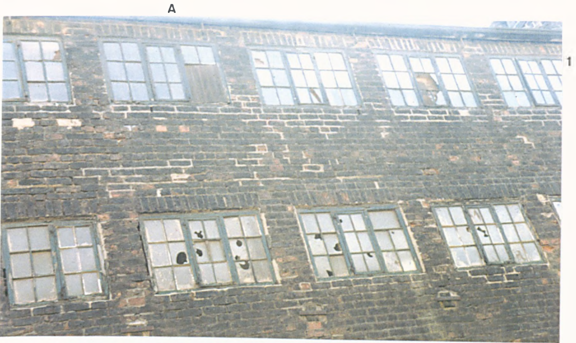
Figure 28b: Traditional cutlery workshop windows that open outwards. Note the hinges at A1.
