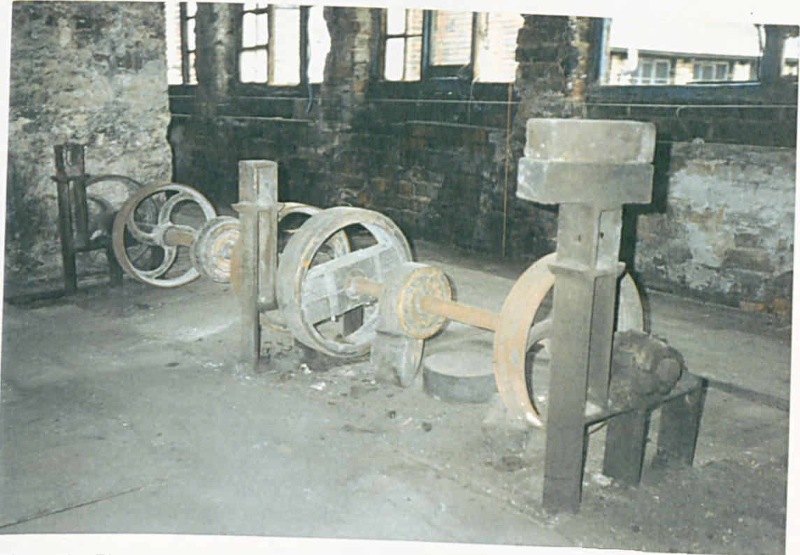
Figure 4a: Photograph by the owner of line shafting before it was removed from Kendal Works (1994).
