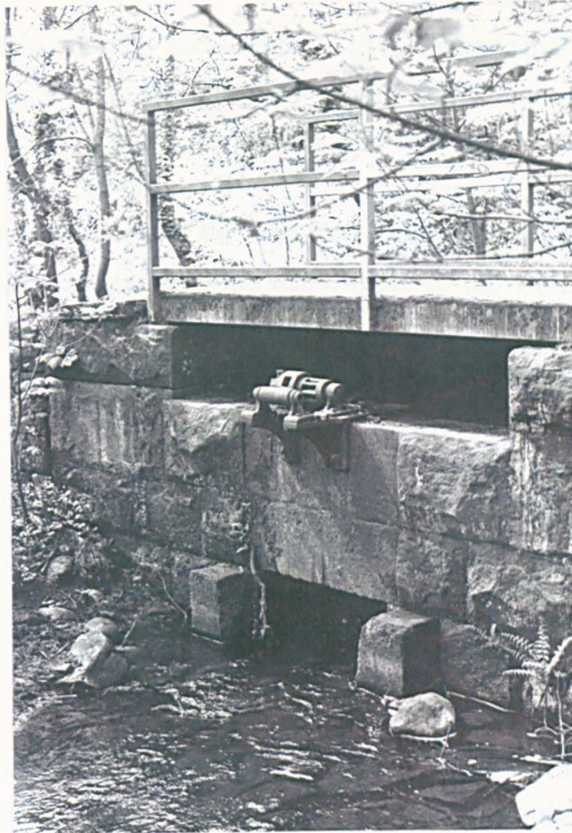
Figure 5b: Entry to head goit at Little London Wheel (Rivelin) showing the ratchet system used from the nineteenth century for lifting the sluice.
