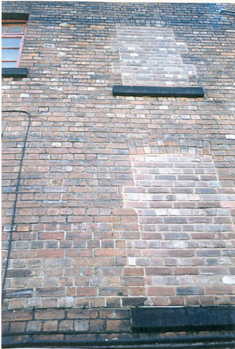
Figure 7d: English bond used in the construction of Alpha Works, Carver Street
