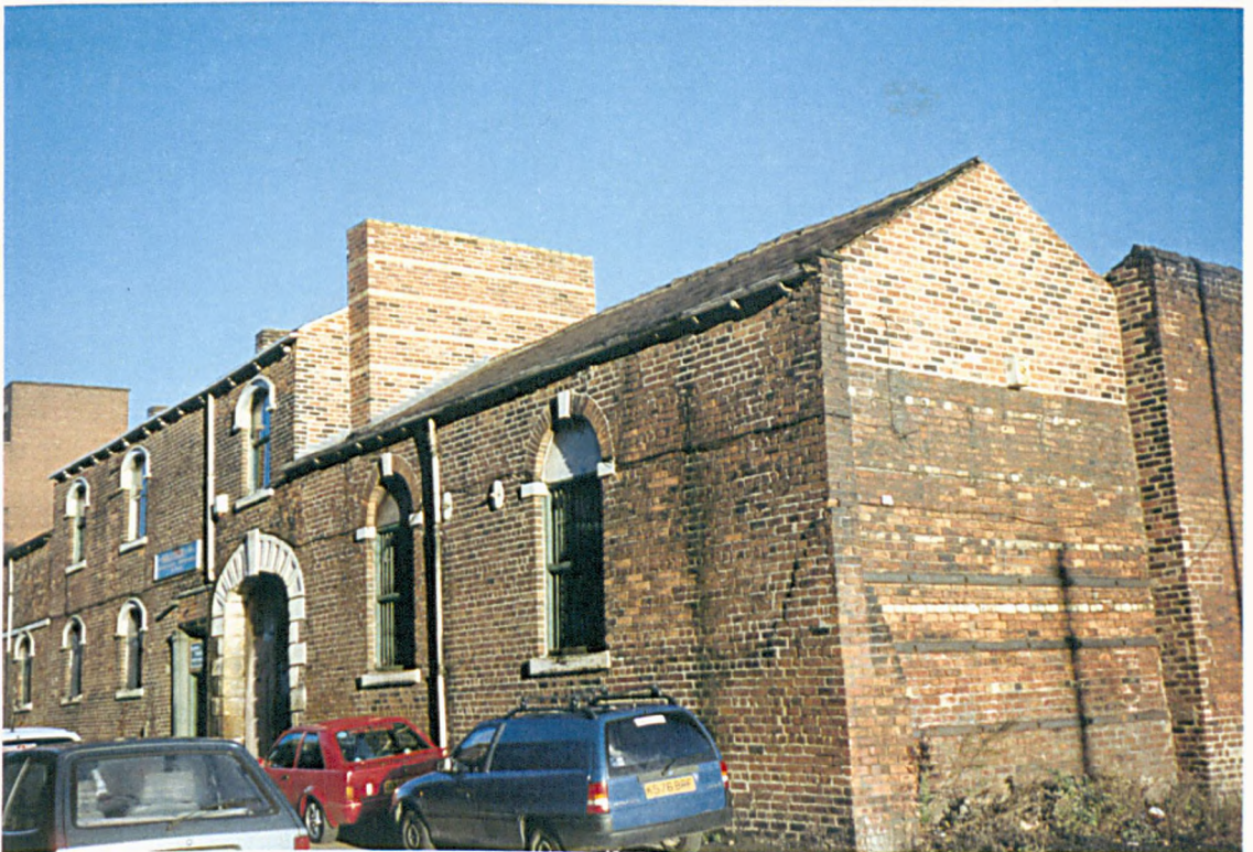
Figure 20: Crucible Stack, Malinda Street.
