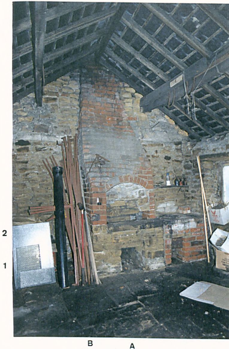
Figure 5b: File Forger's Hearth, Stepping Lane, Grenoside. Note that the chimney breast is stepped and constructed of brick, whilst the base is of stone. It is also possible to see the ash hole (A1) and hole for tuyere (B2) indicating that the bellows were situated to the left of the hearth. On the right is a bowl under which a fire could be lit. This may have been used for melting lead used to make the beds on which the files were cut (see section on file cutting, this chapter).
