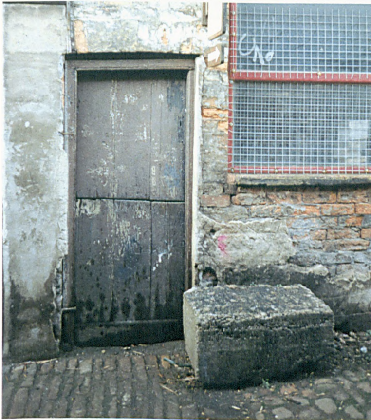
Figure 22a: Example of a Stable or Dutch door at forge in Garden Street.
