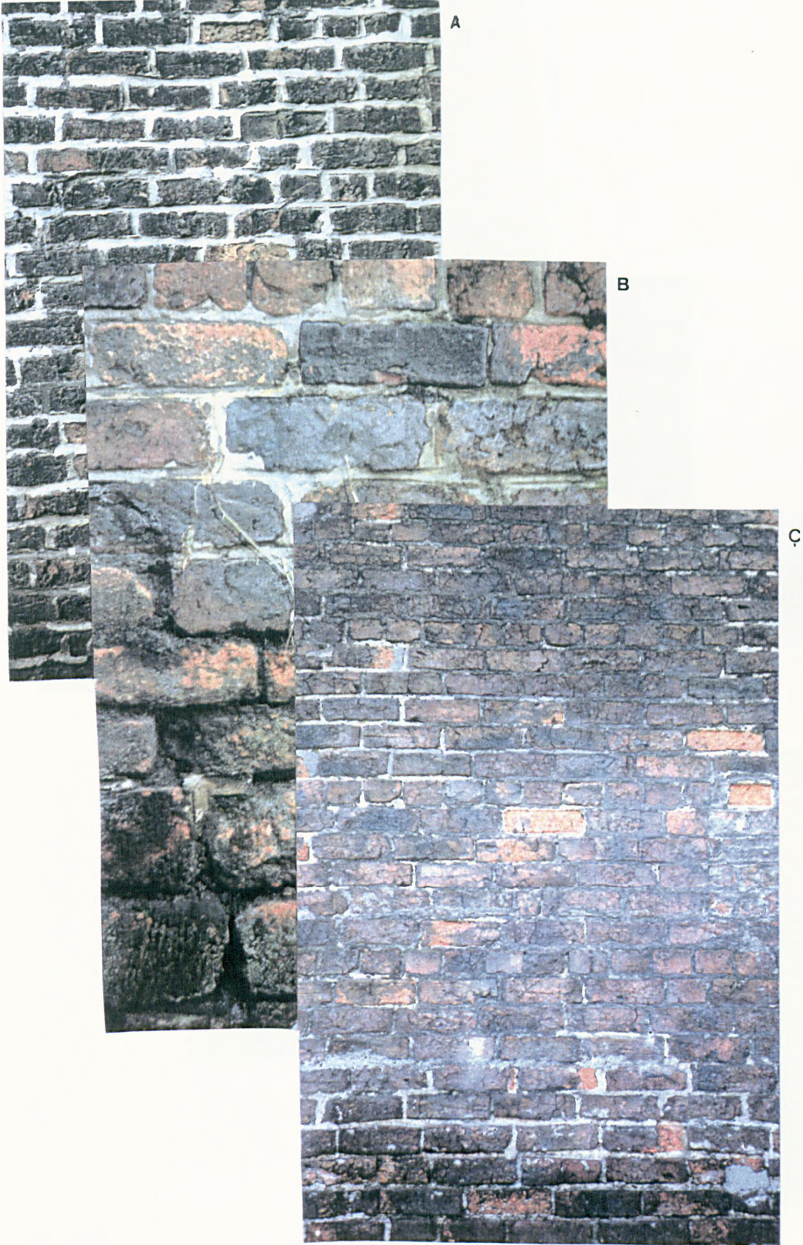
Figure 8: B1 Type Bricks. A: Elliot's 1840 Workshop Block, Sylvester Street, B: 50 Garden Street, C: Kendal Works, workshop block, Carver Lane.
