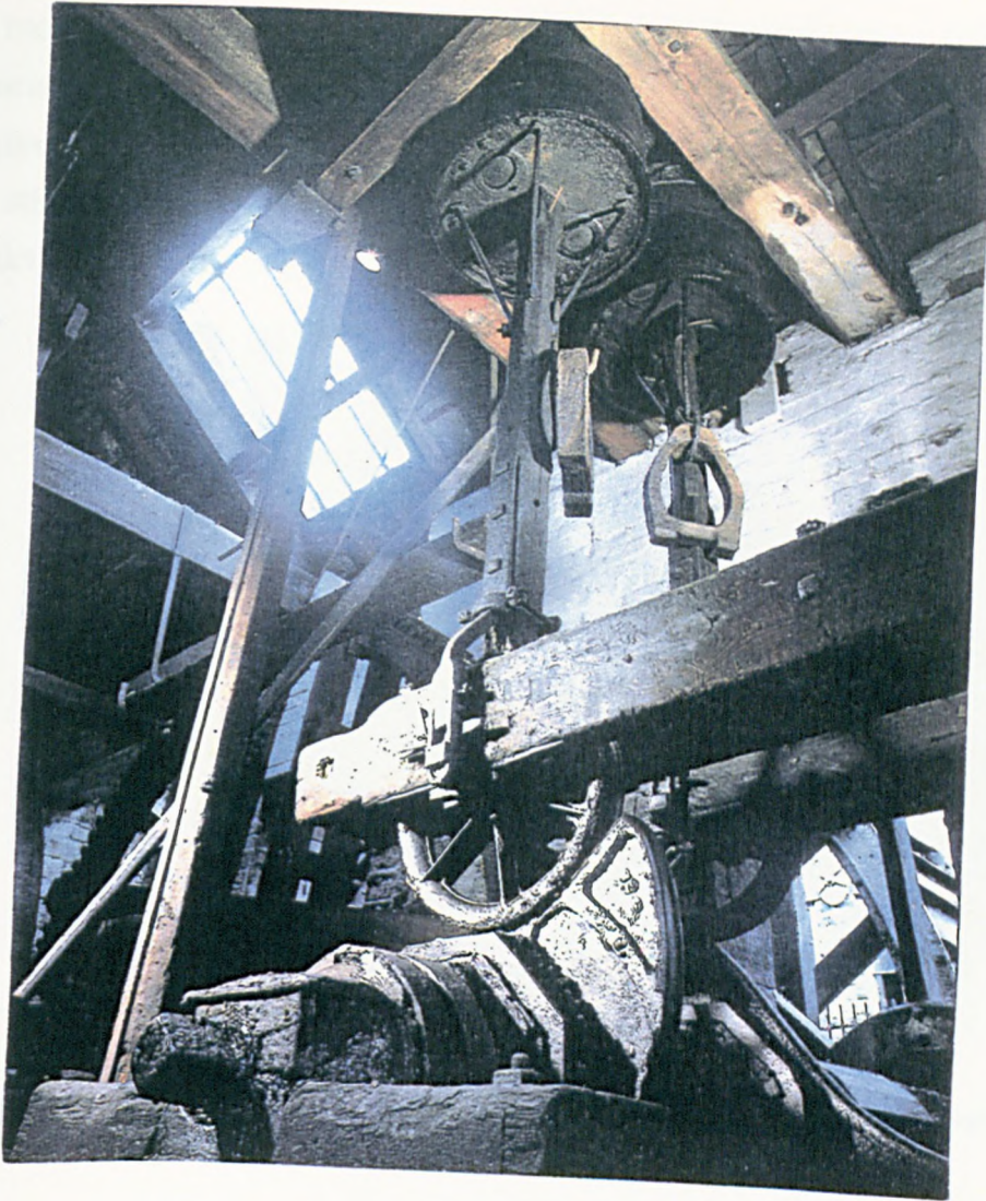
Figure 22: The operation of the tilts by a cam system at Abbeydale (Sheffield Museum Publications 1985) 1: ride on triple acting cams, 2: fitted directly to water wheel shaft, 3: cylinders in which pistons are working.
