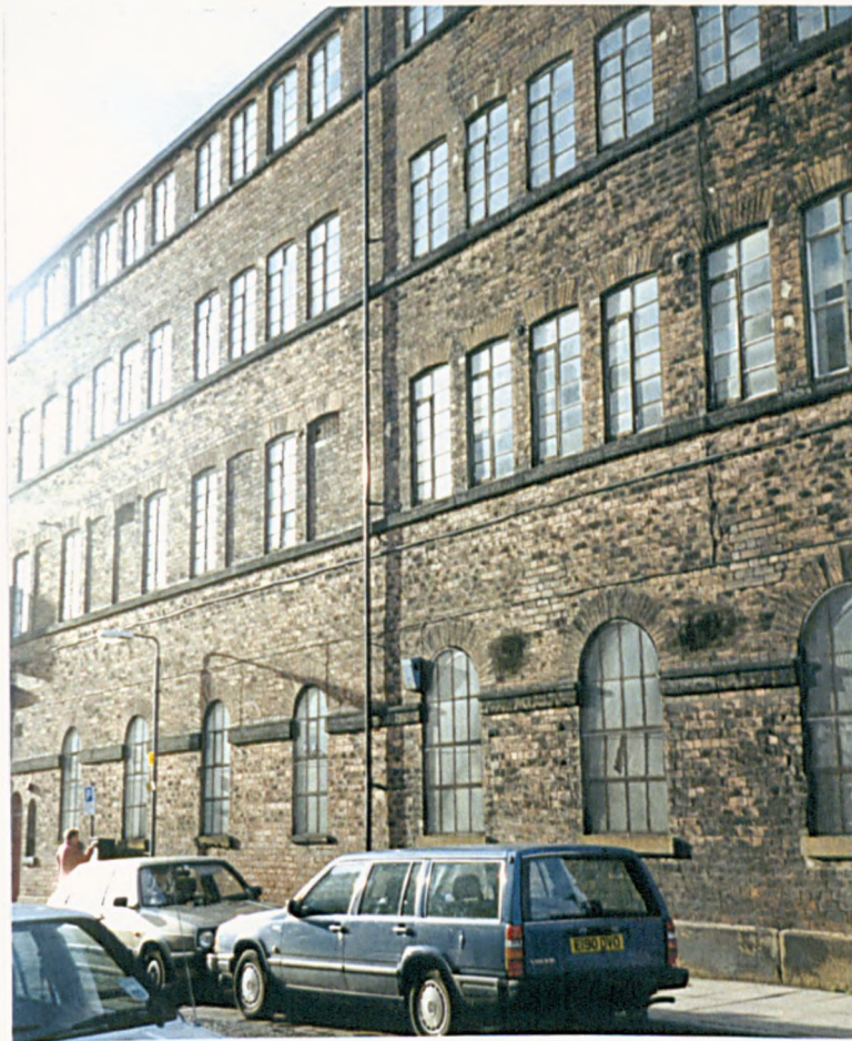
Figure 29a: Frontage of Butcher's Wheel showing the larger windows (A1) used for the room which housed the engine.
