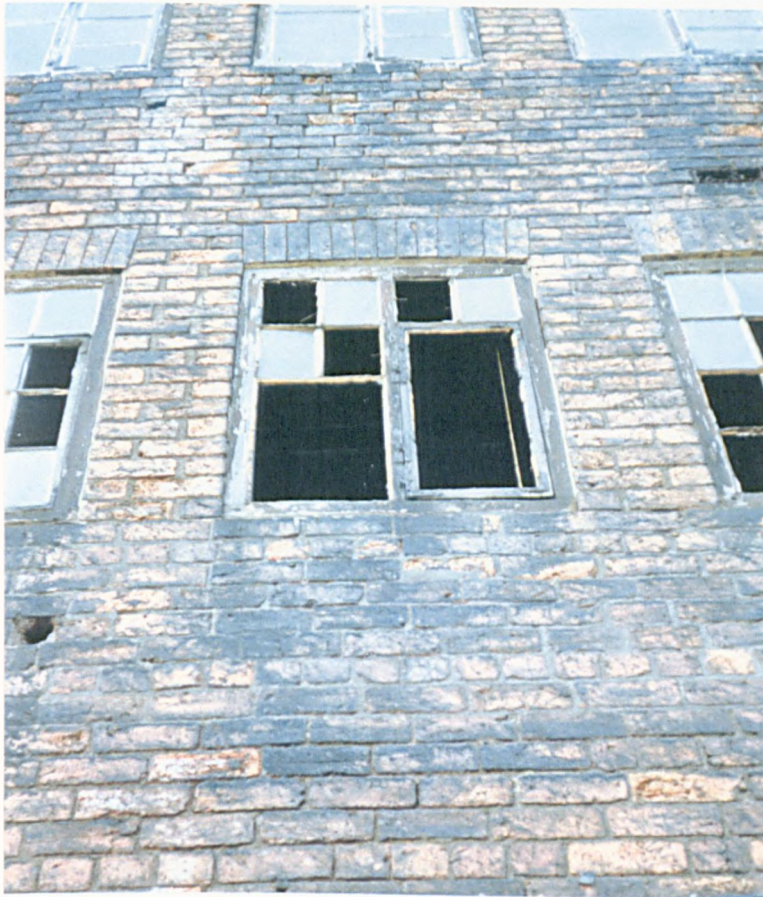
Figure 30a: Decoration is rarely found above the typical windows of the cutlery workshop. The example above shows vertical bricks above windows in Egerton Street.
