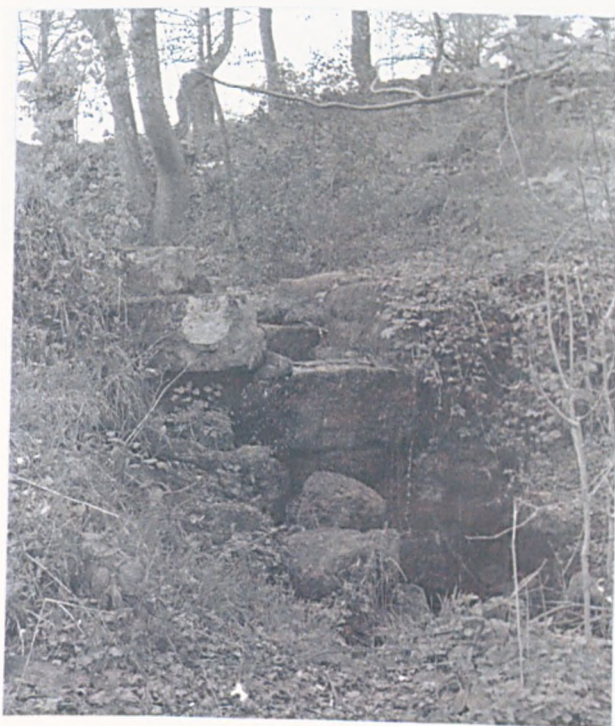
Figure 12a: When the structure of the pentrough does not survive the location can be established from the surviving masonry as at Second Coppice Wheel.
