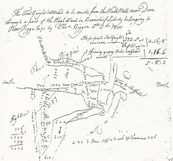
Figure 24a: Digging a Tail goit at Walk Mill (FB87p7)
