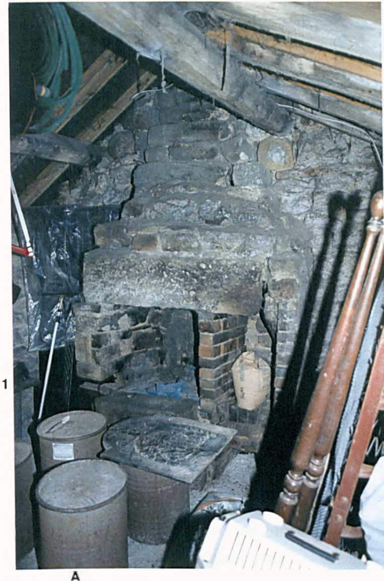
Figure 5a: Scissor forger's workshop, Bingley Cottage, Stannington. This hearth has a stone breast and lintel. Note the hole for the tuyere at A1. The space on the right-hand side of the hearth may have been used for tempering the blades.
