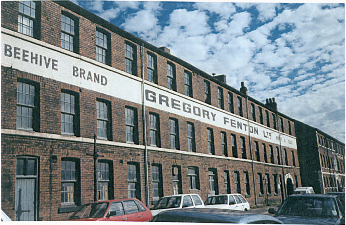
Figure 36a: Office and Packing Shop windows at Gregory Fenton's Beehive Works, Milton Street.
