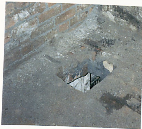
Figure 34: Possible power transmission shaft hole at Butcher's Wheel
