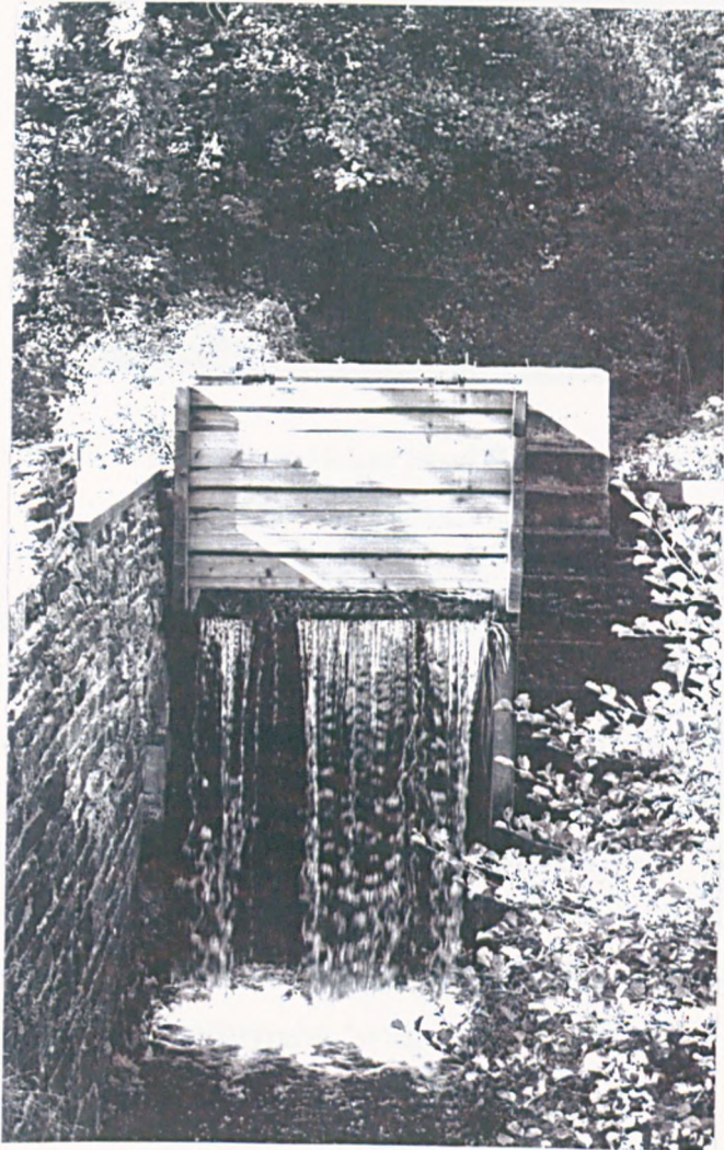
Figure 11a: Pentrough restored at Rowell Bridge (Loxley)
