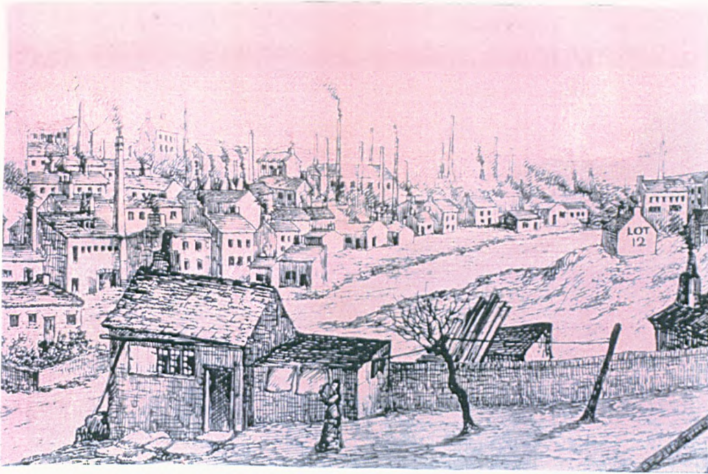
Figure 18: Topham's View of Sheffield from the site of the Midland Station 1866 shows the tall hearth chimneys to be found attached to some workshops in the town.
