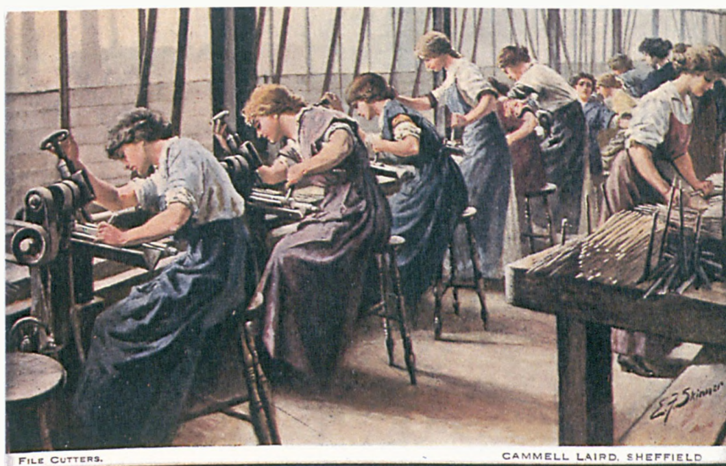
Figure 30: Machine File Cutting at Cammell Laird's.
