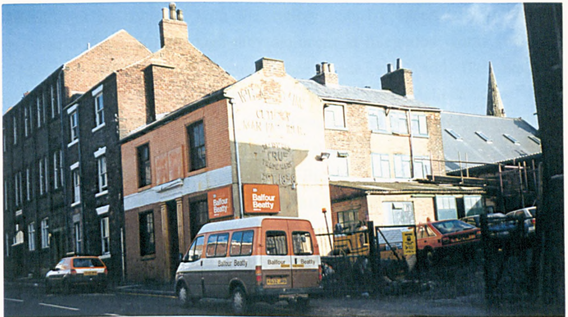
Figure 17b: Fireplace chimney on Wm. Bocking's Workshop, Gell Street
