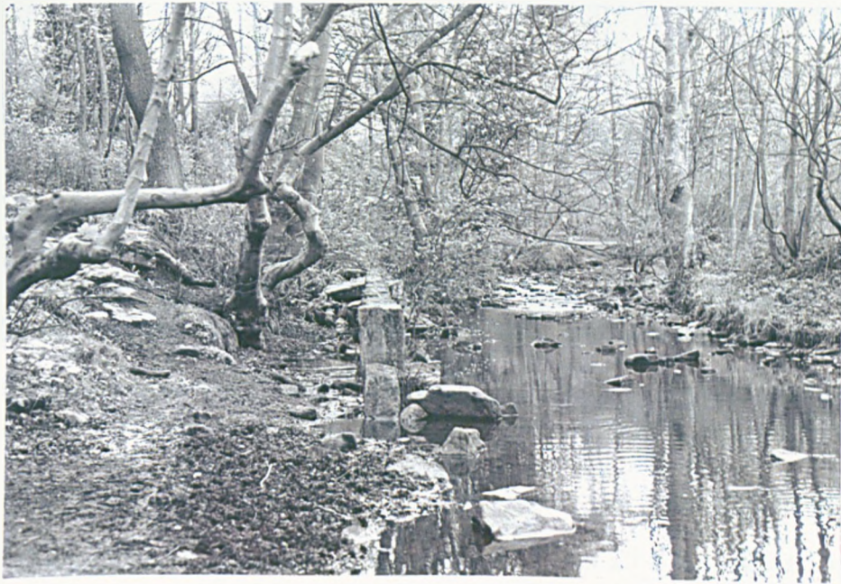
Figure 23a: Upstream view of extended tail race at Holme Head Wheel where large ashlar blocks separate the tail race (A1) from the Rivelin (B2).
