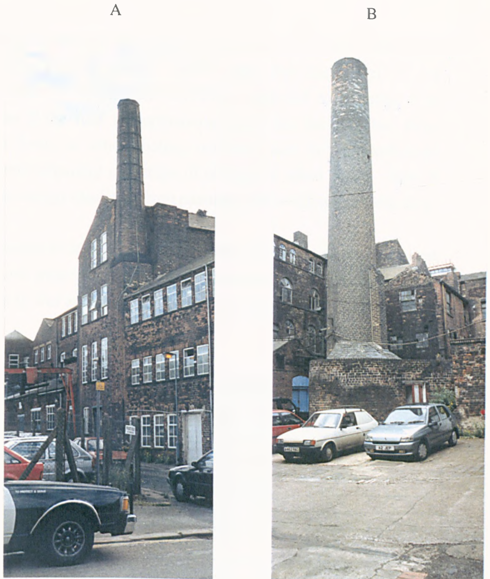
Figure 21: Chimneys for engines at A) Eye Witness Works and B) Butcher's Wheel
