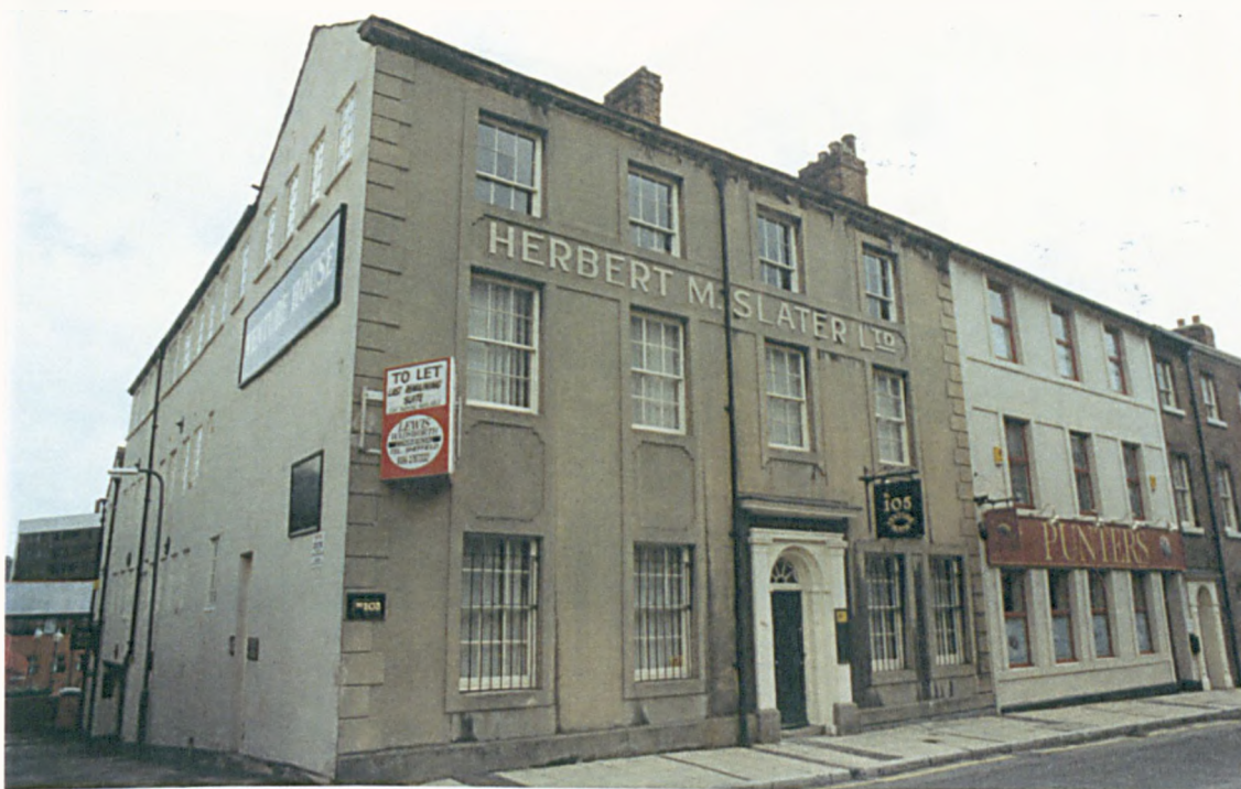
Figure 3a: Slater's Venture Works, Arundel Street. Note the Town-house frontage and the addition of the workshops to the rear. (1995)
