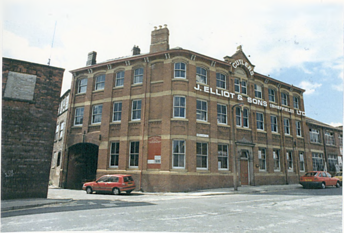
Figure 5: Elliot’s Sylvester Works, Arundel Street. One of the few examples of ‘constructional polychromy’ used on an industrial building in Sheffield. Note the ashlar course at the top of each storey and the use of layers of bricks (A1) to create different textures.
