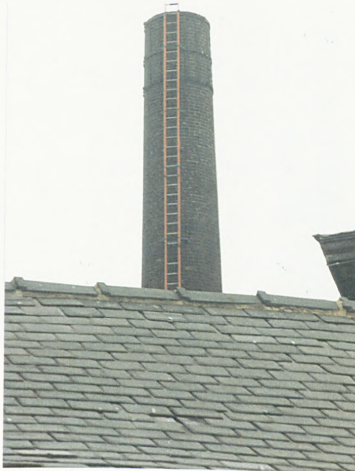
Figure 6b: Chimney at Cornish Place.
