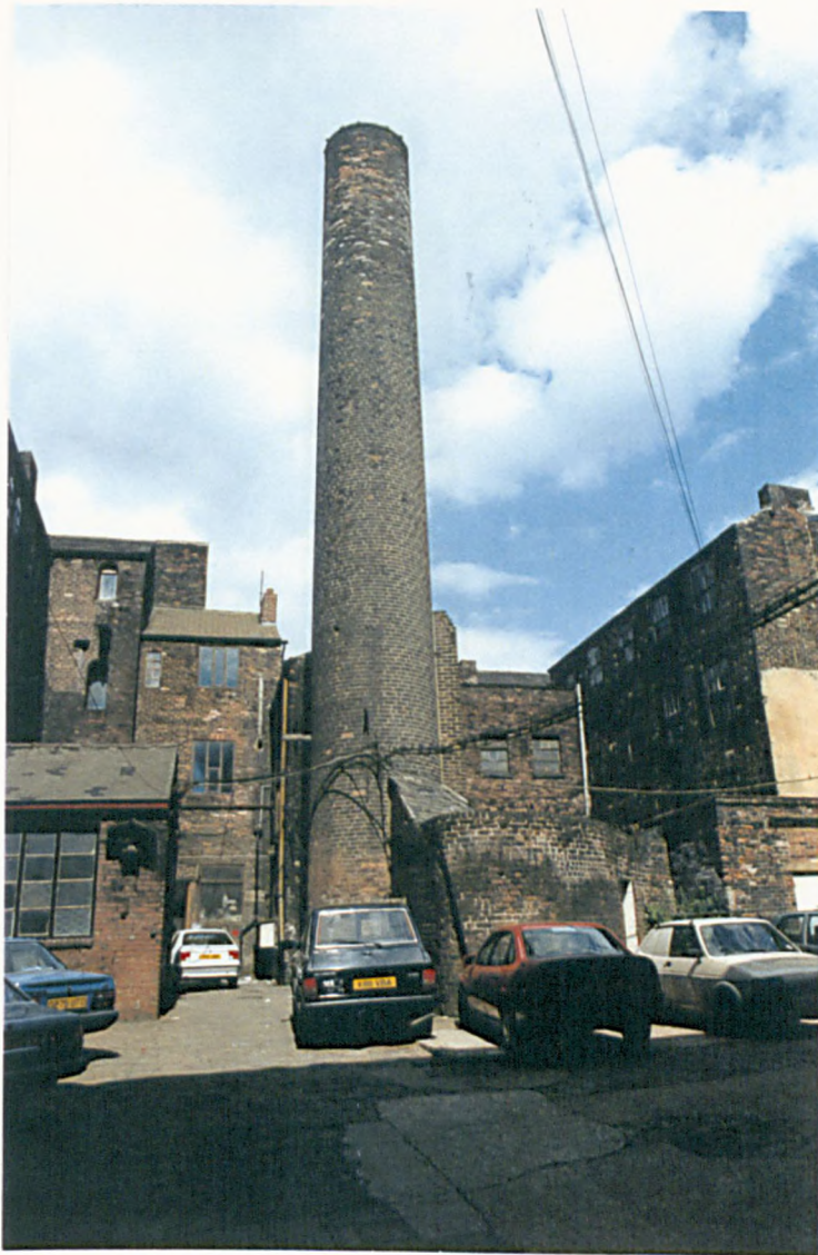
Figure 6a: Chimney at Butcher's Wheel, Arundel Street. Like that at Cornish Place (6b) it has retained its functional simplicity in keeping with other structures in the complex.
