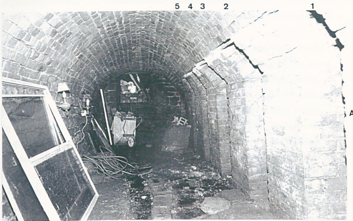
Figure 22: Cellar beneath a five-hole crucible furnace that may have belonged to the Tingles, in Back Lane, Grenoside. (Note the Ash pits at A 1-5)
