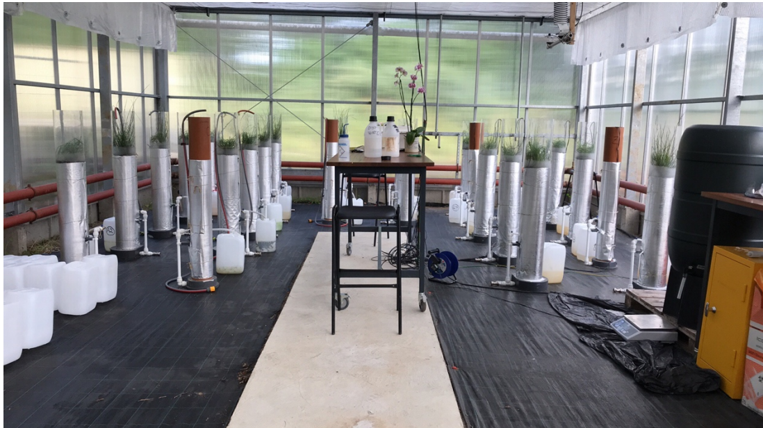
Figure 3-5 Panoramic view of the neo-built biofiltration facility. On the left, columns have accessory pipes for hydraulic conductivity assessment. On the right, columns installed with sensors. Water was prepared in a 250 litre water butt. Samples were collected every two weeks swapping outlet tanks with clean ones (bottom left)
